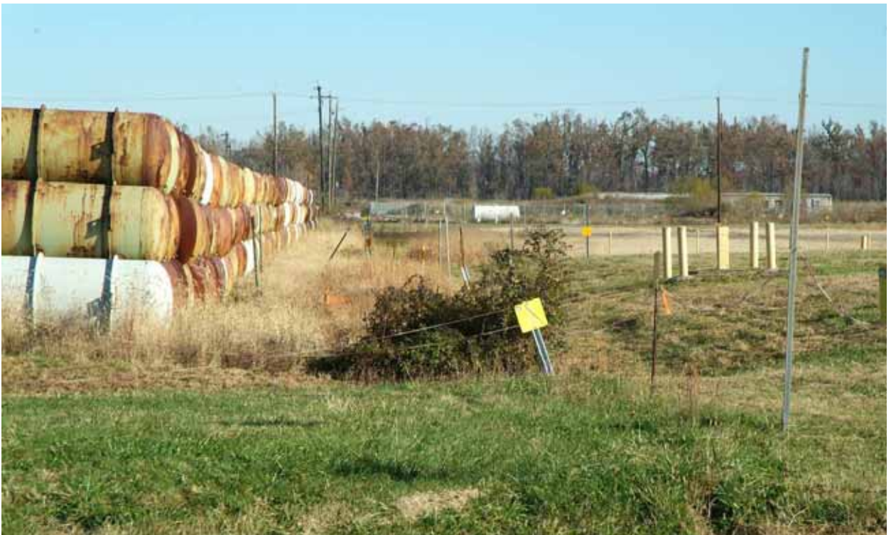
Figure E.20. Outfall 015 EU07 11-12-09 (Before)
