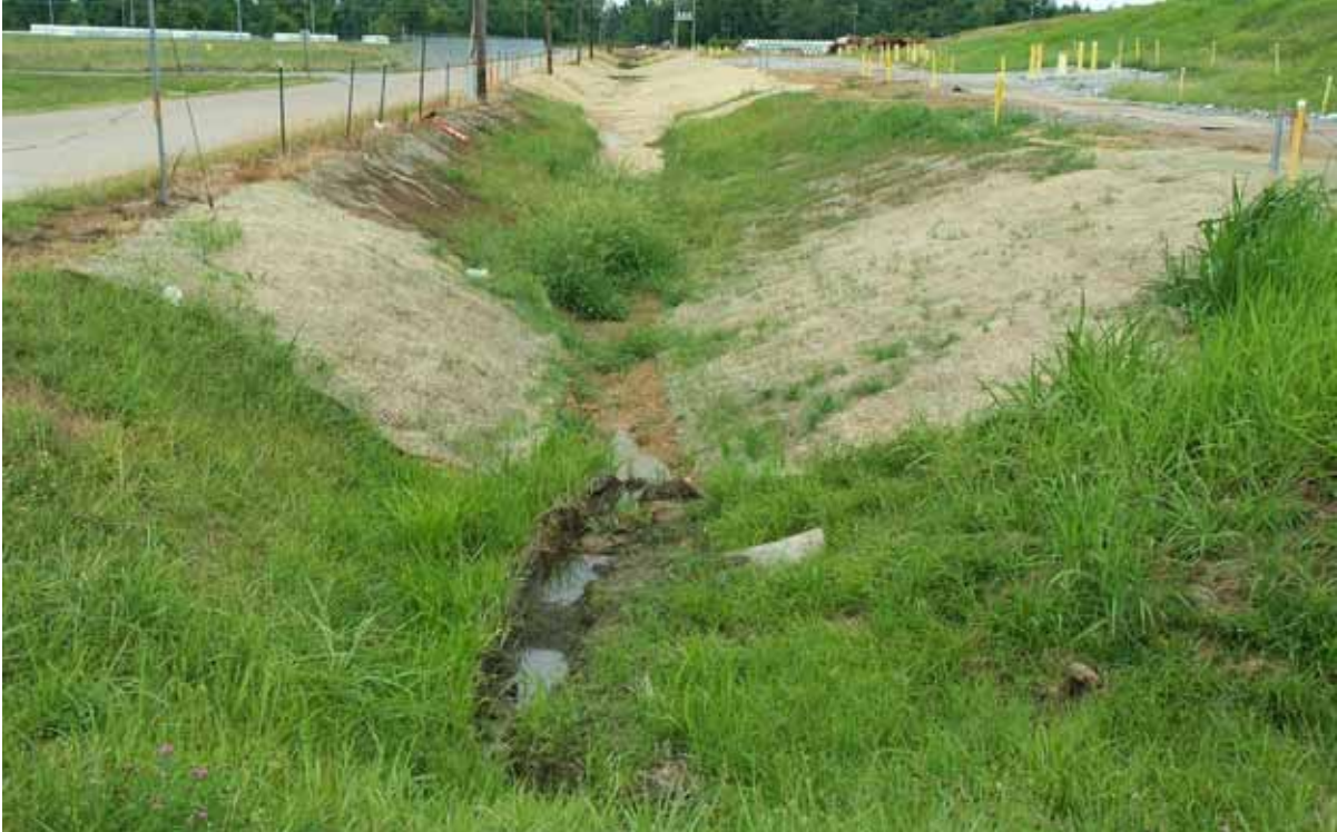
Figure E.27. Outfall 015, EU 03 07-12-10 (After)
