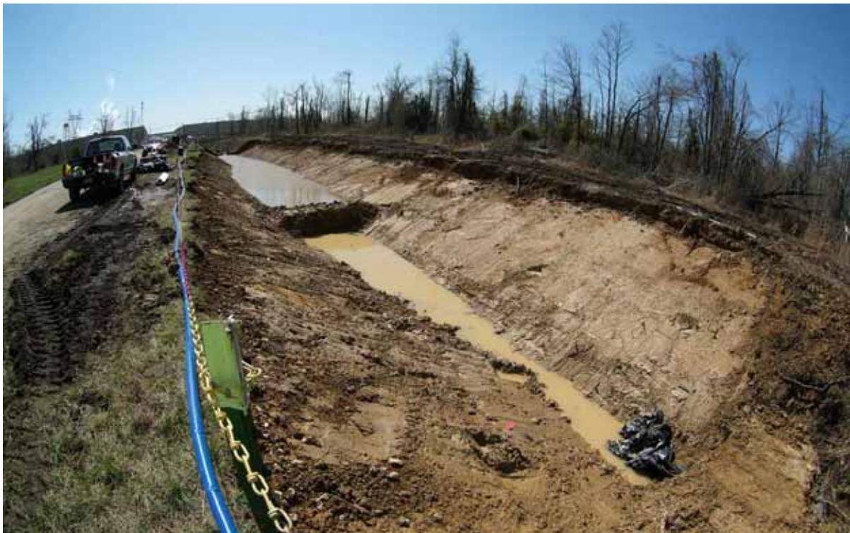
Figure E.36. North-South Diversion Ditch Section 3 EU 02 3-26-10 (During)
