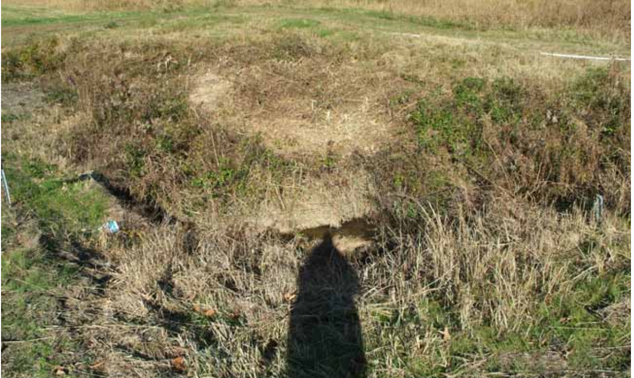
Figure E.33. North-South Diversion Ditch Section 3, EU 03 11-12-09 (Before)
