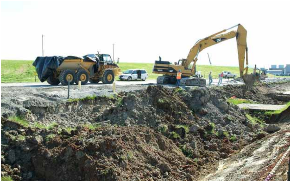
Figure E.22. Outfall 015, EU 03 04-28-10 (During)
