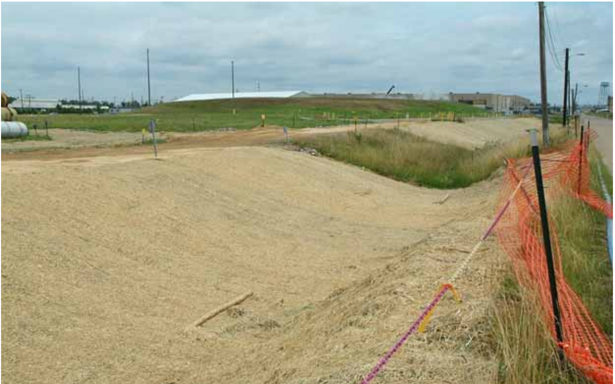
Figure E.26. Outfall 015, EU 02/03 07-12-10 (After)
