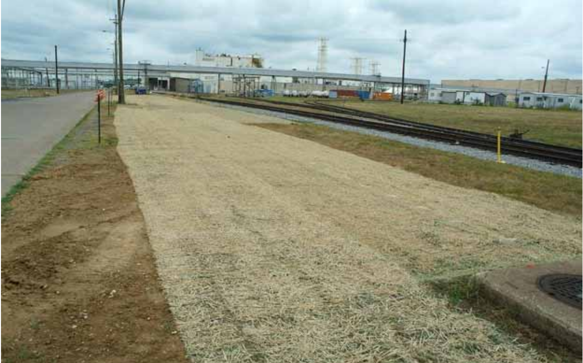
Figure E.9. Outfall 010 07-12-10 (After)
