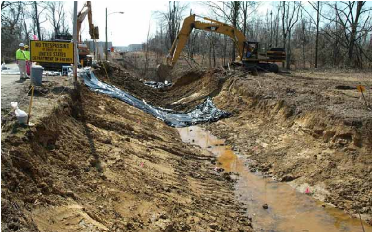
Figure E.38. North-South Diversion Ditch Section 3 EU 03 03-26-10 (During)
