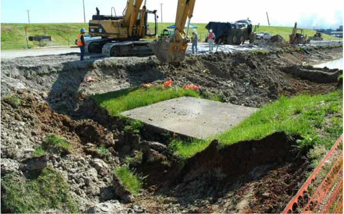
Figure E.23. Outfall 015, EU 03 04-28-10 (During)
