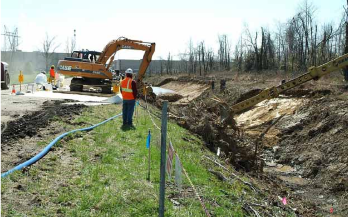
Figure E.37. North-South Diversion Ditch Section 3 EU 02/03 03-26-10 (During)
