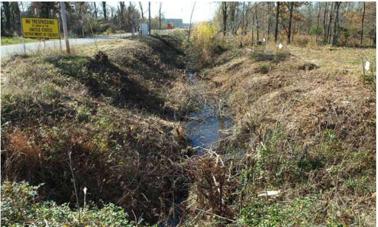
Figure E.32. North-South Diversion Ditch Section 3, EU 03 11-12-09 (Before)
