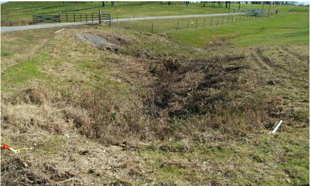
Figure E.34. North-South Diversion Ditch Section 3, EU 03 11-12-09 (Before)
