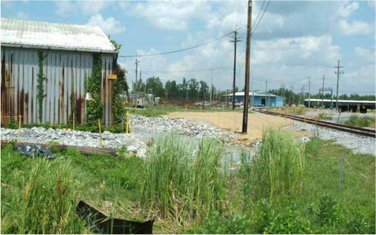
Figure E.6. Outfall 001 07-22-10 (After)
