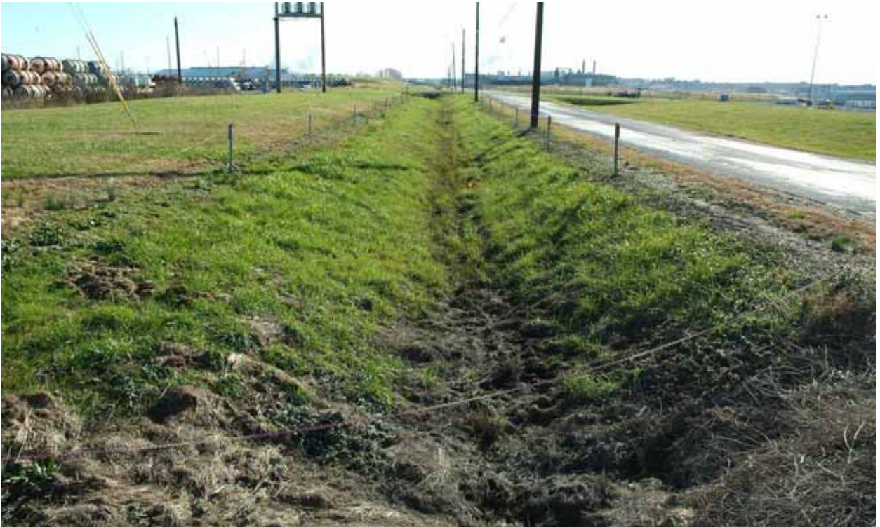
Figure E.14. Outfall 015, EU02 11-12-09 (Before)
