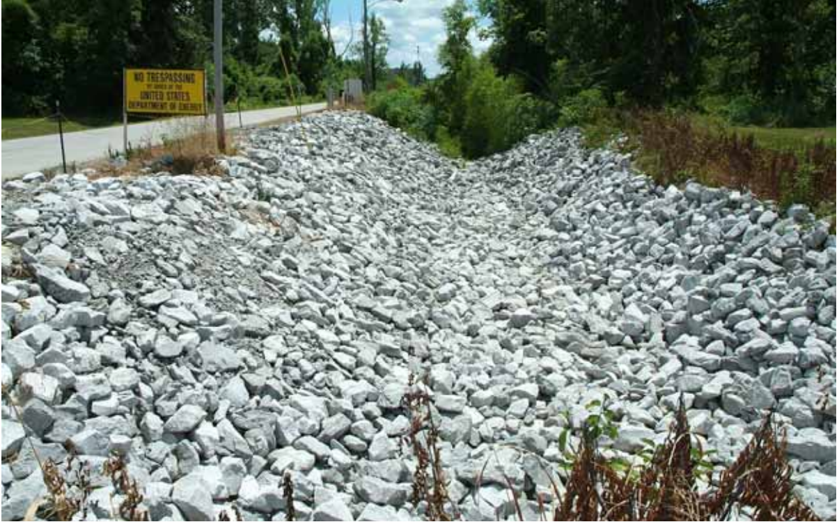
Figure E.41. North-South Diversion Ditch Section 3 EU 03 07-13-10 (After)
