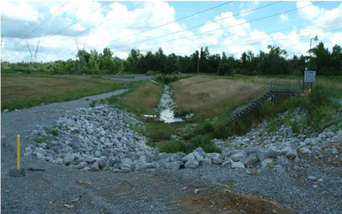
Figure E.12. Outfall 011 07-12-10 (After)
