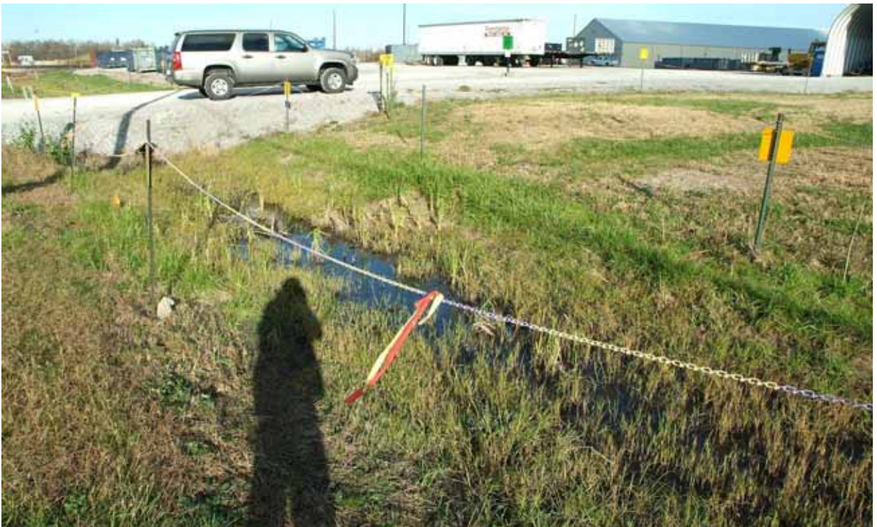
Figure E.18. Outfall 015 EU04 11-12-09 (Before)
