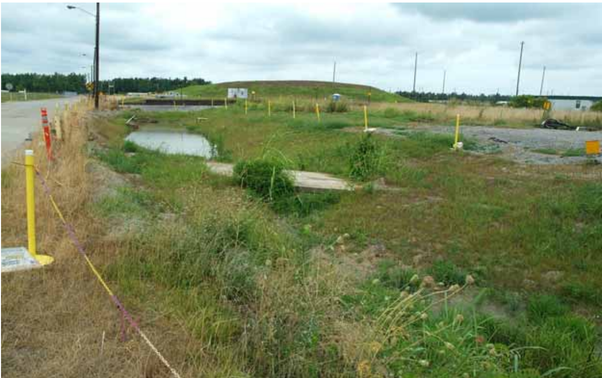
Figure E.28. Outfall 015, EU 04 07-12-10 (After)
