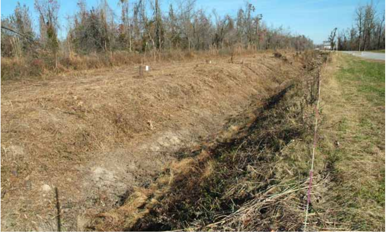
Figure E.31. North-South Diversion Ditch Section 3, EU 02 11-12-09 (Before)
