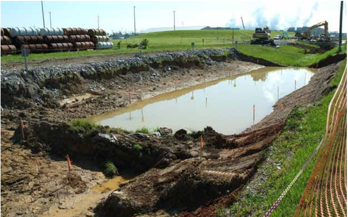
Figure E.24. Outfall 015, EU 02 04-28-10 (During)
