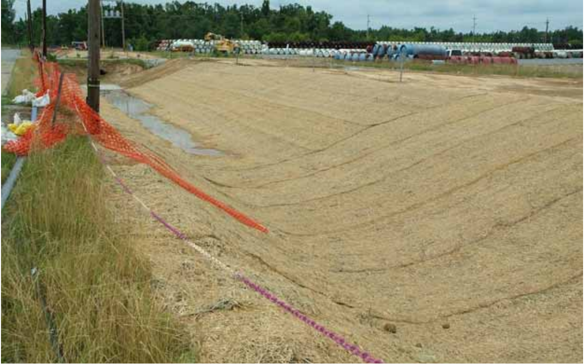
Figure E.25. Outfall 015, EU 02 07-12-10 (After)
