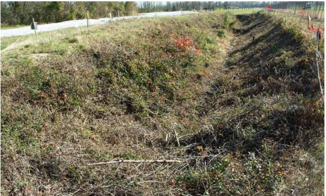
Figure E.30. North-South Diversion Ditch Section 3, E U01 11-12-09 (Before)
