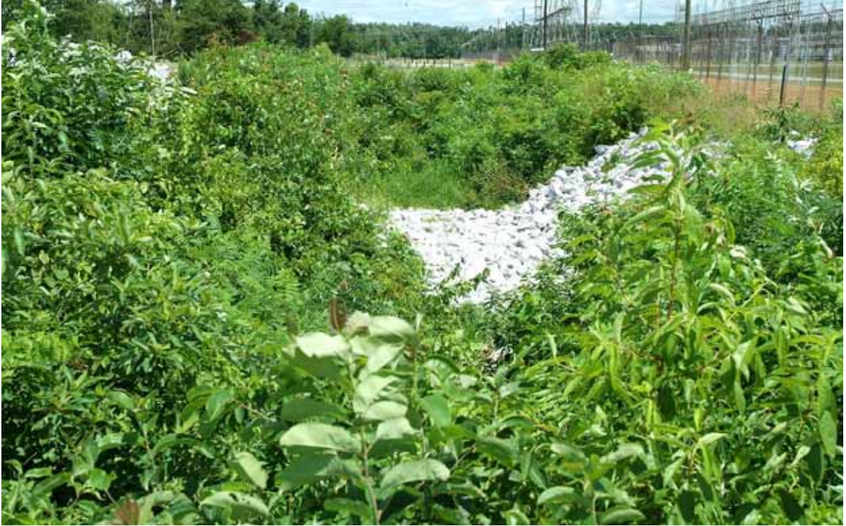
Figure E.39. North-South Diversion Ditch Section 3 EU 01 07-13-10 (After)
