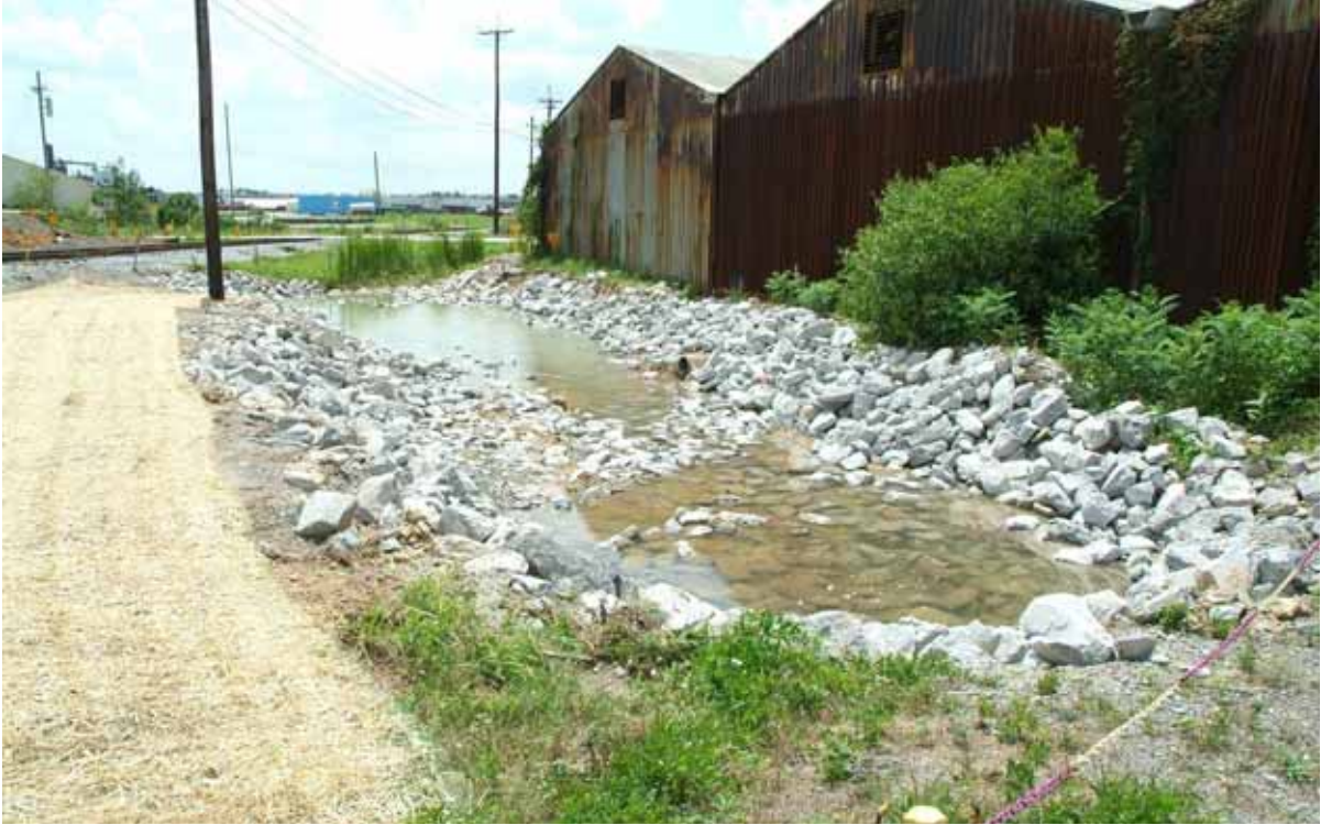
Figure E.5. Outfall 001 07-22-10 (After)
