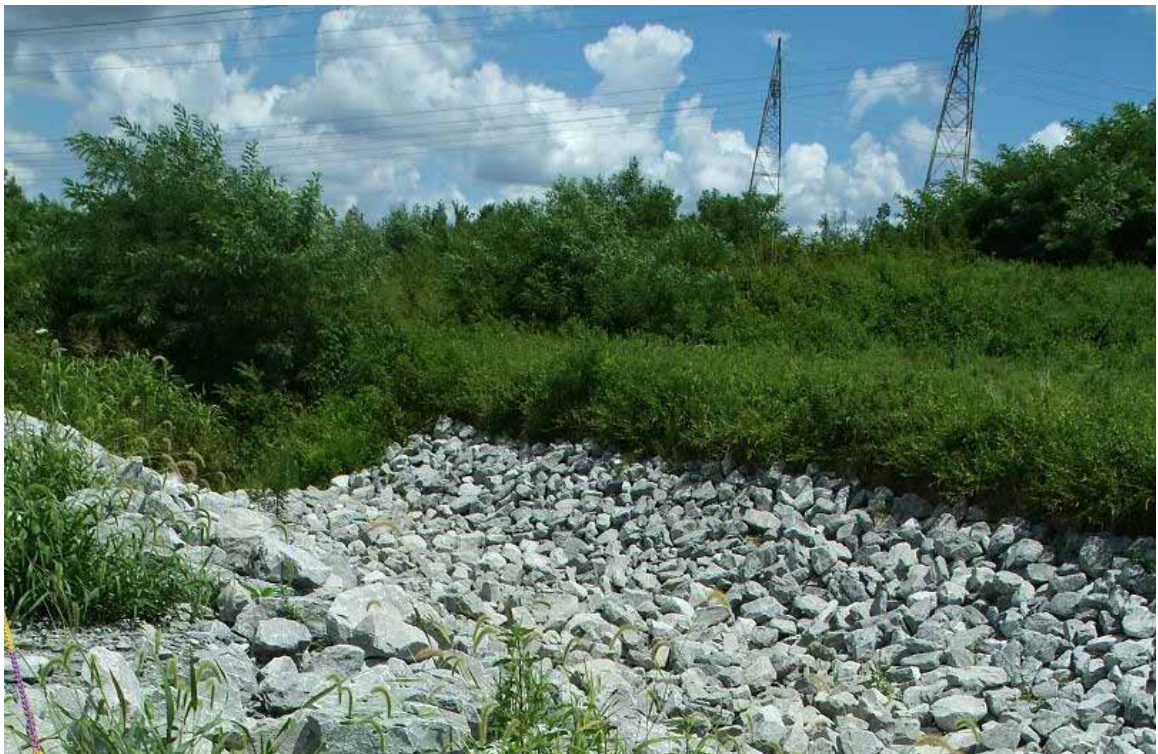
Figure E.42. North-South Diversion Ditch Section 5 07-13-10 (After)
