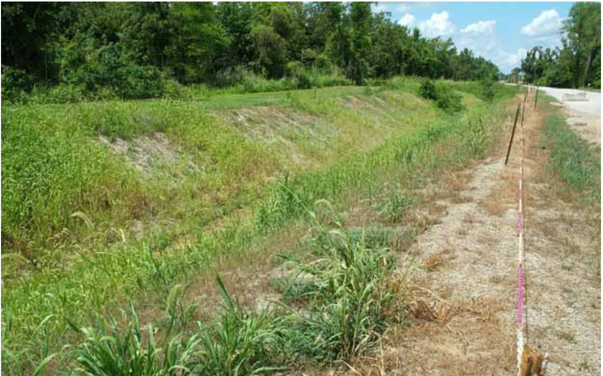
Figure. E.40. North-South Diversion Ditch Section 3 EU 02 07-13-10 (After)
