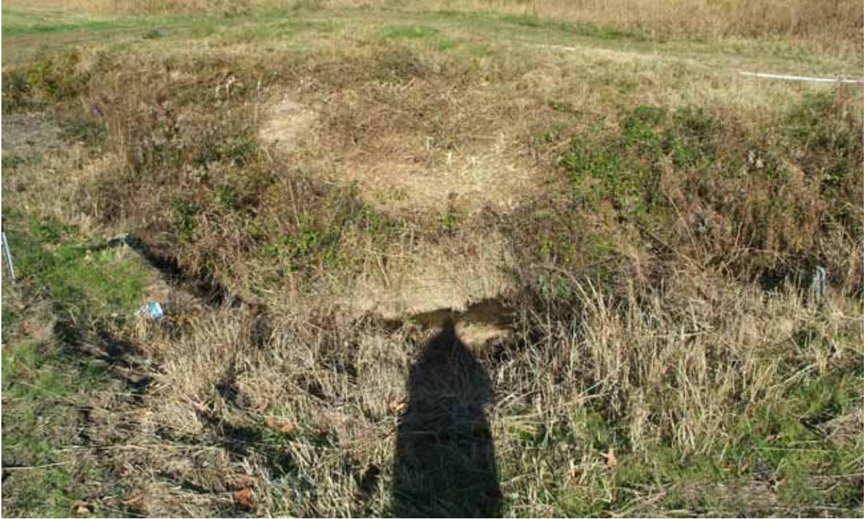
North-South Diversion Ditch Section 3, EU 03 11-12-09 (Before)
