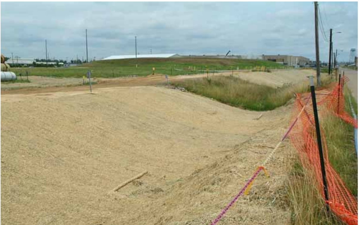
Outfall 015, EU 02/03 07-12-10 (After)
