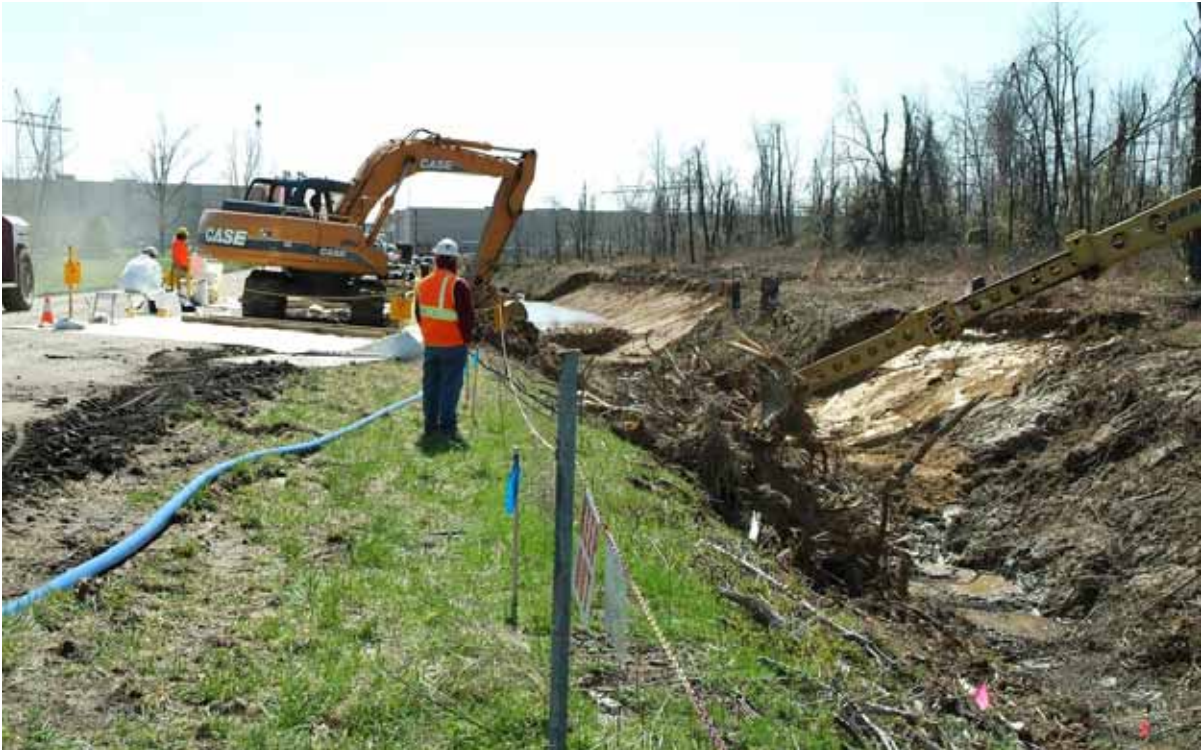
North-South Diversion Ditch Section 3 EU 02/03 03-26-10 (During)
