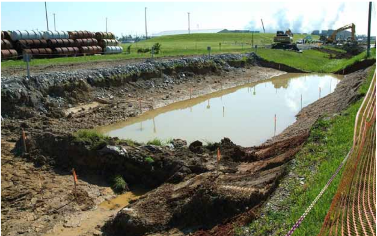
Outfall 015, EU 02 04-28-10 (During)
