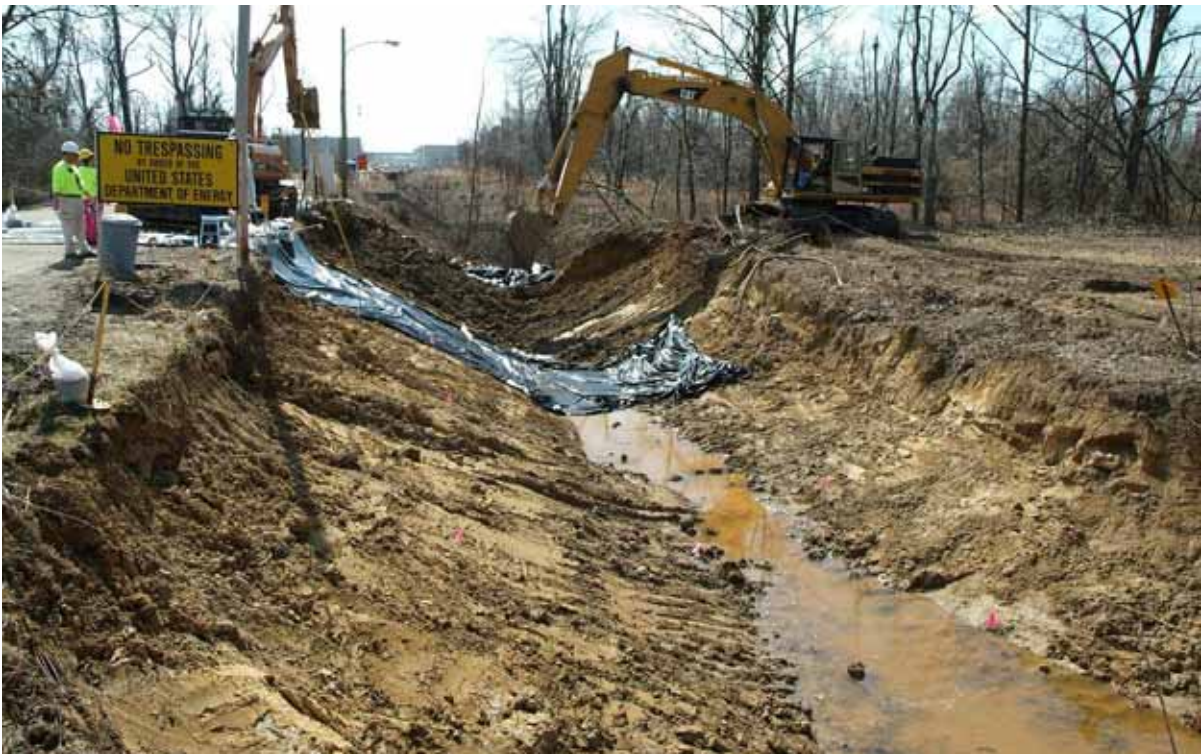
North-South Diversion Ditch Section 3 EU 03 03-26-10 (During)
