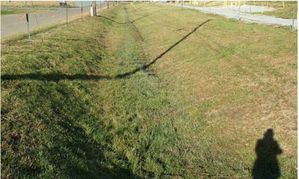
Outfall 015 EU03 11-12-09 (Before)
