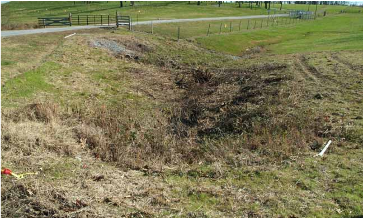
North-South Diversion Ditch Section 3, EU 03 11-12-09 (Before)
