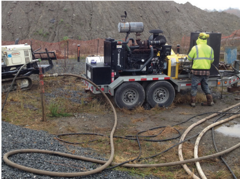
A Jetstream Waterblaster high-pressure water pump used to perform the water jetting phase of DPT jet injection.
