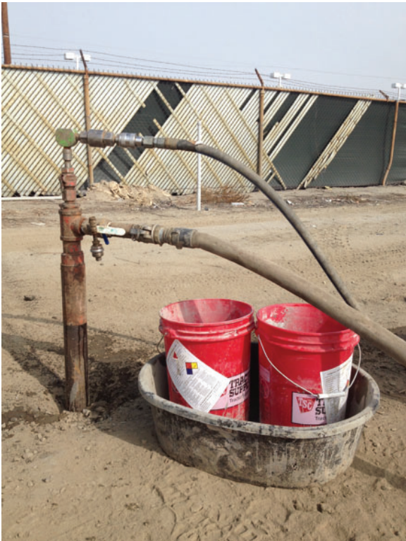
A DPT jet injection wellhead with a high-pressure water line (top) and a slurry injection line (bottom).
