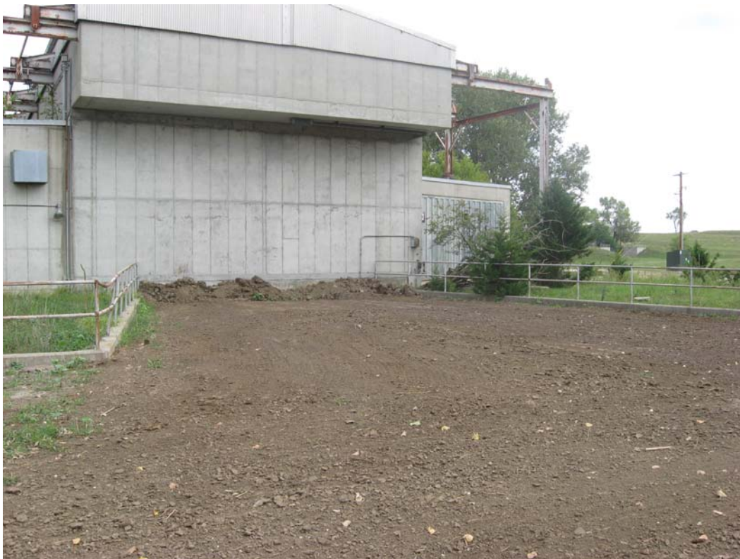
Photo 2: LSB2 Flame Pit Area After Site Preparation Activities
