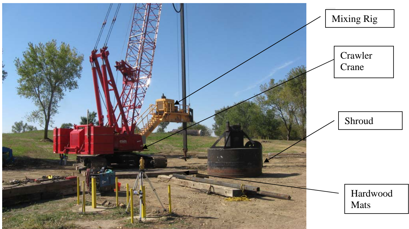
Photo 3: Mixing Rig, Crawler Crane, and Shroud
