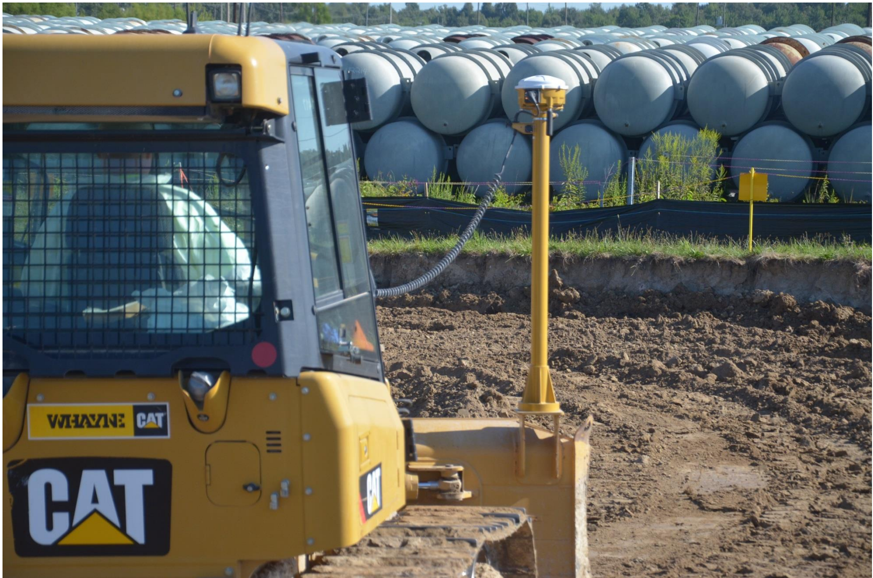
Figure 16. Bulldozer Mounted with AccuGrade™ System (Looking North on August 14, 2014)
