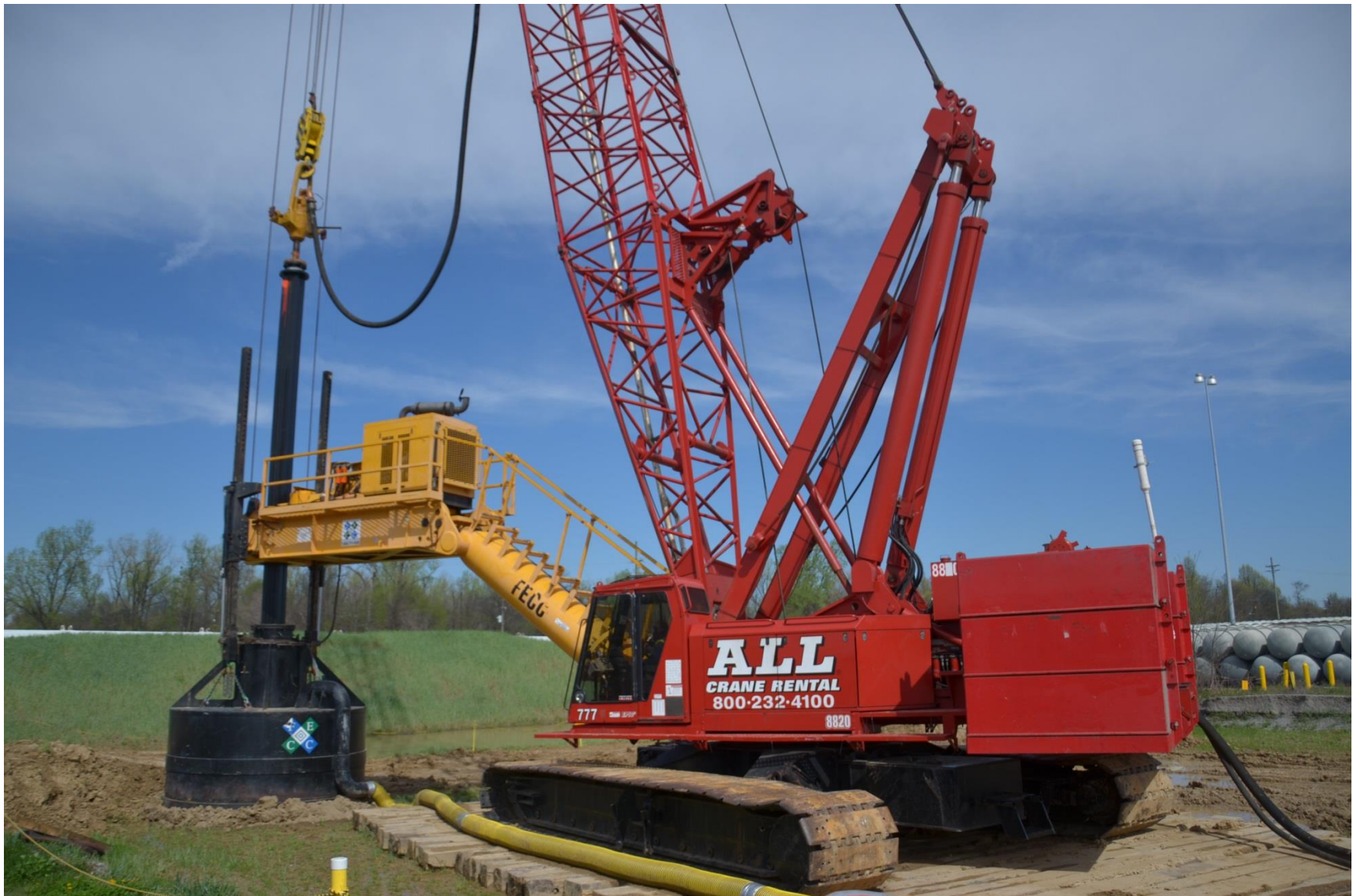
Figure 28. Manitowoc Crane and Soil Mixing Assembly
