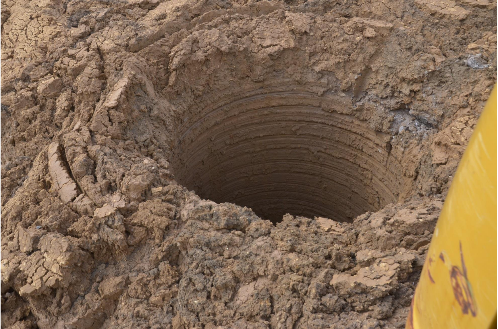
Figure 24. Ejection of Soil Column Resulting from Release of Energy (Soil Burp)
