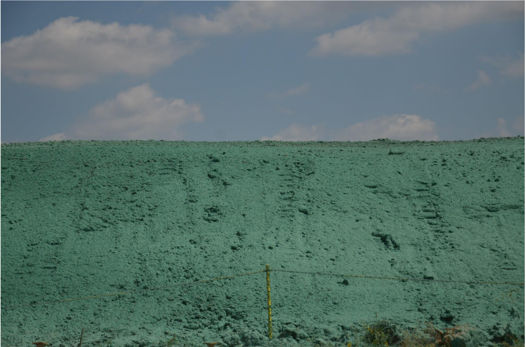
Figure 18. Soil Staging Pile after Hydromulching
