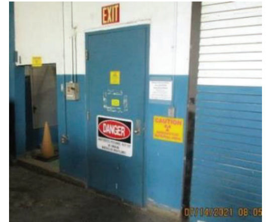
South Door Interior Entry to 90-Day Accumulation Area
