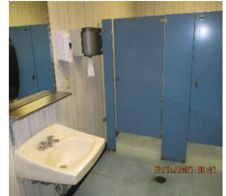
Floor Drain - Restroom
