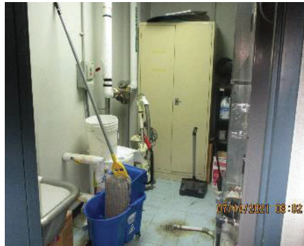
Floor Drain – Mechanical/Electrical/Janitorial Room
