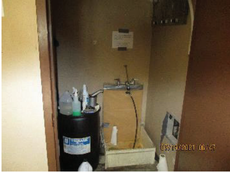
East Storage Room
