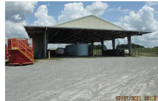
C-752-C Facility Photo: 7/2021
