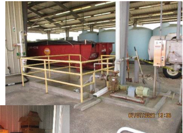
Sump Pit #1 and Frac Tank and Poly Tanks
