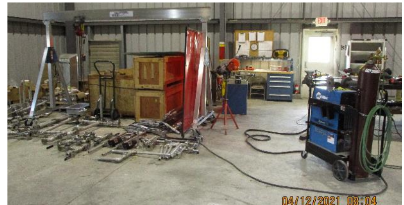
Hot Work Area for Pipe Fabrication
