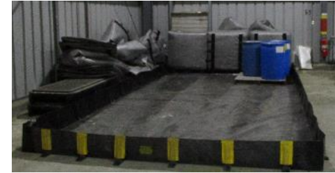
Containment for Propylene Glycol Storage Area
