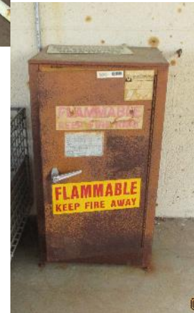
Flammable cabinet - contains wasp spray, hornet spray, and other types of aerosol sprays
