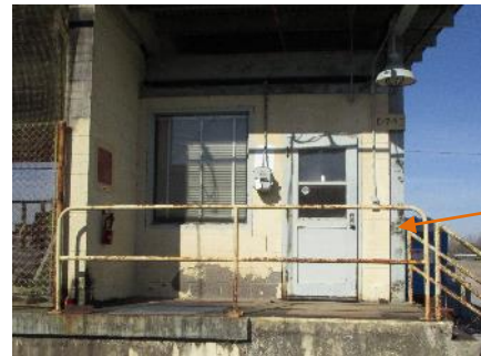
Enclosed Office – North End
