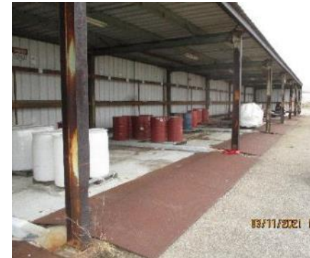
View North to South
