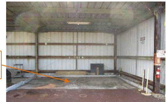
Bay 7 –South End (Former Decontamination Pad)
