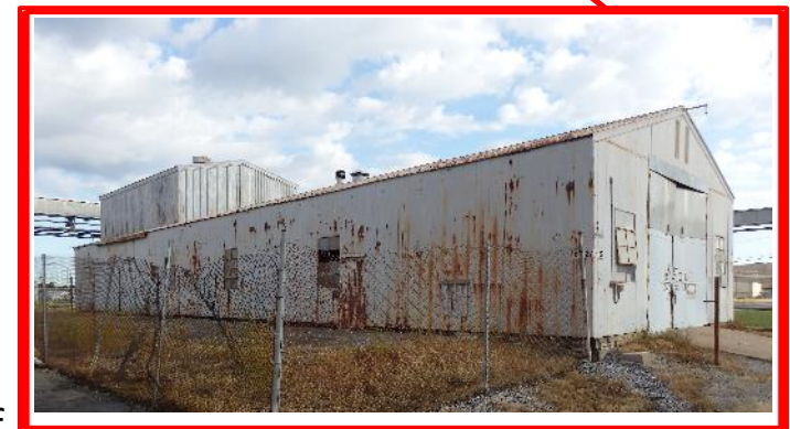
C-727 Facility Photo: June, 2020
