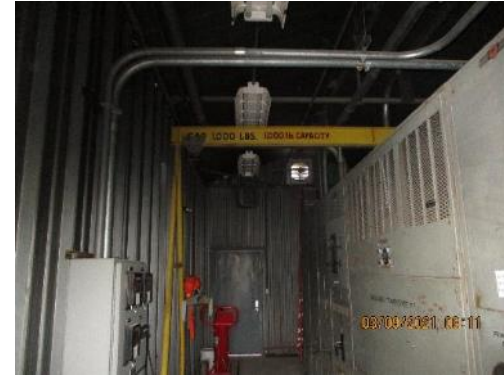
Interior View of C-720-D
