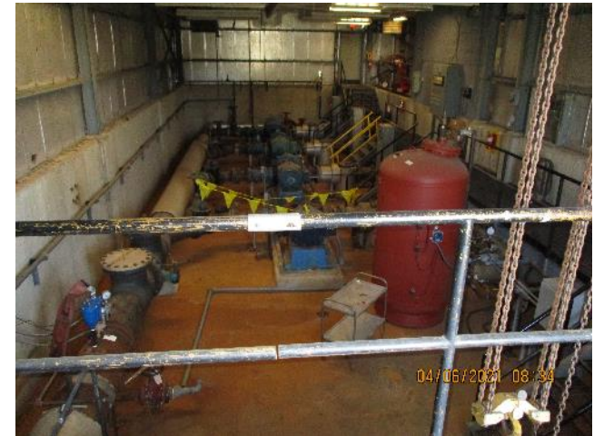
Pump House Section - Subgrade
