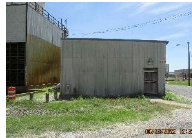
C-631-4 – Blending Pump House North Side
