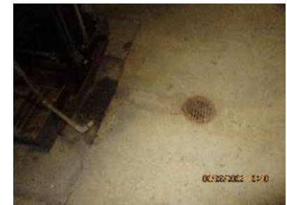
C-631-4 - Floor Drains
