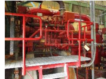
C-631-1 - Center Structure HPFWS Diesel Engine
