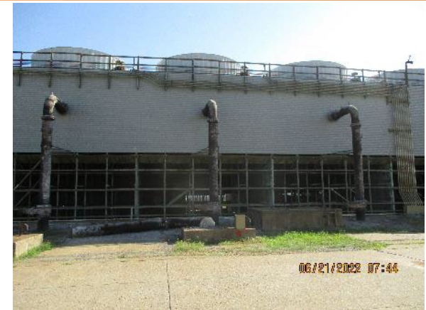
C-631-2 Cooling Tower – South Side
