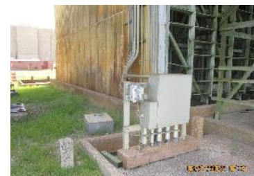
C-631-5 Electric Supply to Fans
