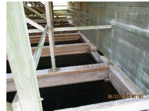
C-631-2 Cooling Tower Basin Interior View
