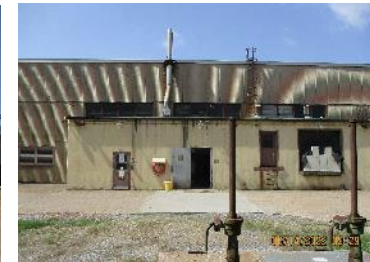
C-631-1 - Pump House North Wing
