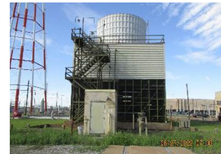
C-631-6 Facility Photos: 6/2022
