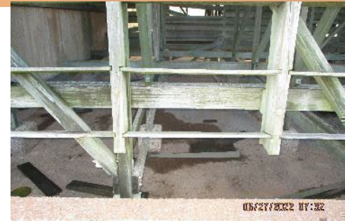
C-631-5 – Structural Frame
