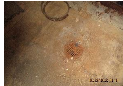
C-631-4 - Floor Drains
