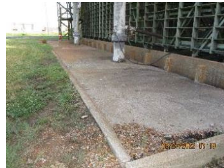
C-631-5 – South Side and No. 10 and No. 11 Risers
