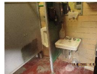
C-631-1 - South Wing Restroom/shower/change area
