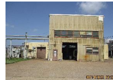
C-631-1 - Pump House Center Structure
