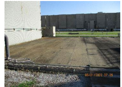
C-631-2 Cooling Tower – East Side (Area Where Cells Formerly Existed)
