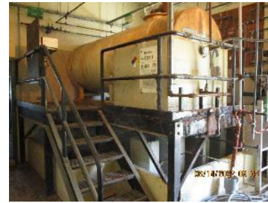
C-631-1 - North Wing Calgon Area
