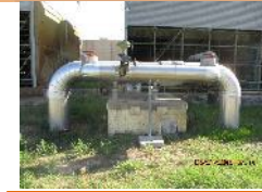
Plant Water Station Vault (Make-up Weir Pit)
