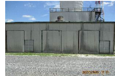
C-631-4 – Blending Pump House West Side
