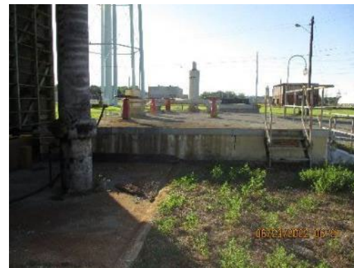
C-631-3 - Pump House (Firewater) West Side
