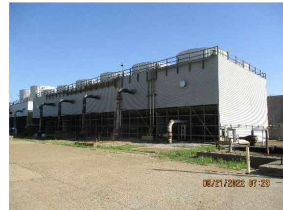
C-631-2 Cooling Tower – South Side
