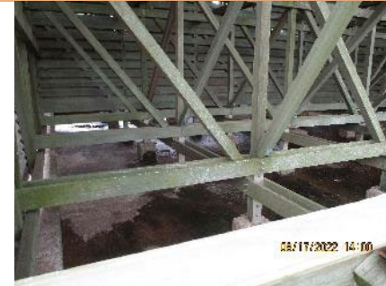
C-631-6 – Structural Frame
