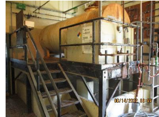
C-631-1 North Wing Diked Area Beneath Corrosion Inhibitor Tanks
