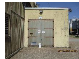
C-631-1 - North Wing Entry to Chlorine Room
