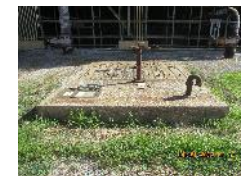
Hot Water Bypass Vault (Valve Vault E)
