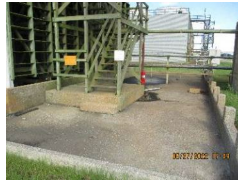
C-631-6 – North Stairway
