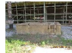
Return Cross Over Vault
