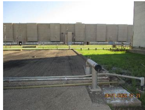
C-631-2 Cooling Tower Basin East Pad with Withdrawl Connections for Firefighting
