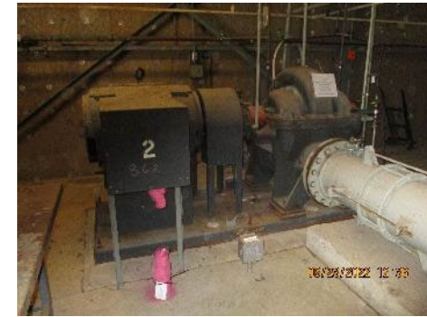
C-631-4 - Skid Frame with Blend Motor and Pump
