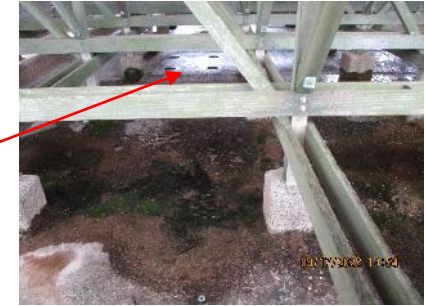
C-631-6 - Top of Basin Slab
