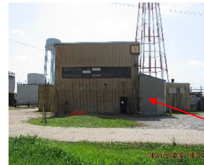
C-631-1 – Lean-to Wing Diesel Tank
