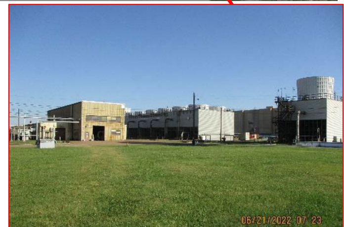
C-631 Cooling Tower Photo: 6/2022
