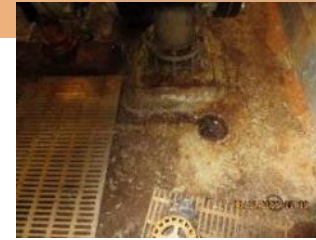
C-631-3 - Floor Drains
