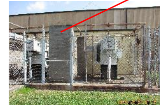
C-631-1 - South Wing External Transformers
