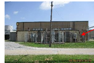
C-631-1 - Pump House South Wing
