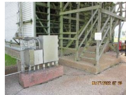
C-631-6 – South Stairway and Electrical Supply to Fan
