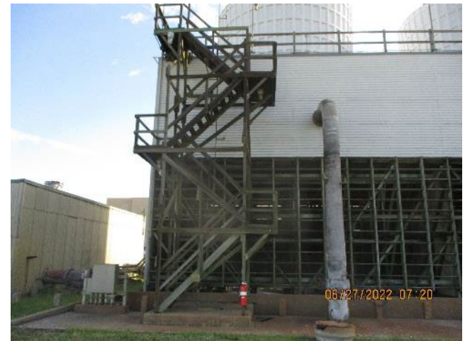
C-631-5 South Side – Riser No. 11
