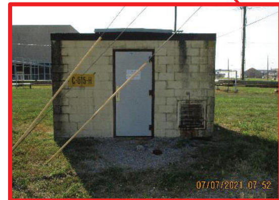
C-615-H Facility Photo: 7/2021
