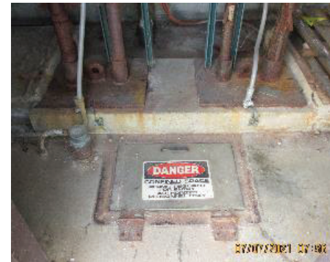
Confined Space Entry to Wet Well
