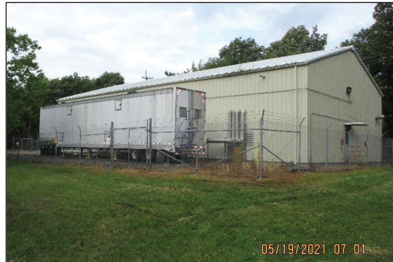
East and North Side of Building (Ion Exchange trailer on east side of C-612)
