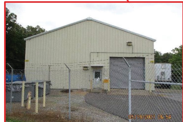
C-612 Northwest Plume Groundwater Treatment Facility Photo: 5/2021
