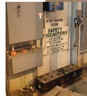
C-607 Facility Photos: 10/2020
