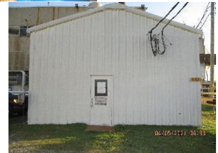
South Side of C-605
