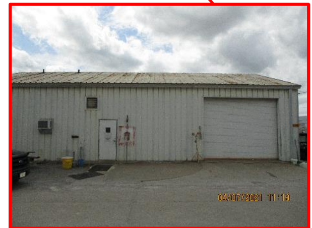
Exterior North Side C-604 Photo: 4/2021
