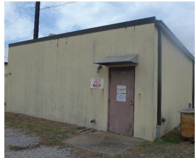
C-303 Facility Photos: 8/2020
