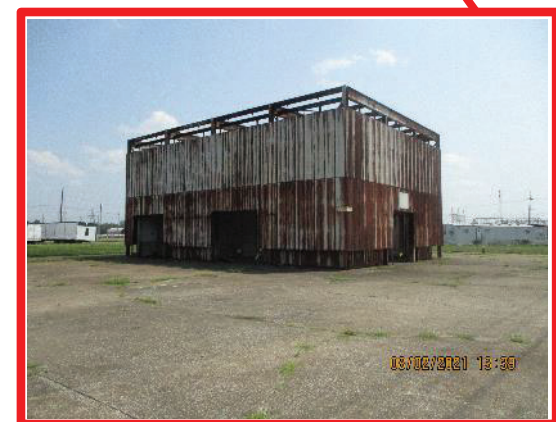
C-301 Fire Training Facility Photo: 8/2021 2
