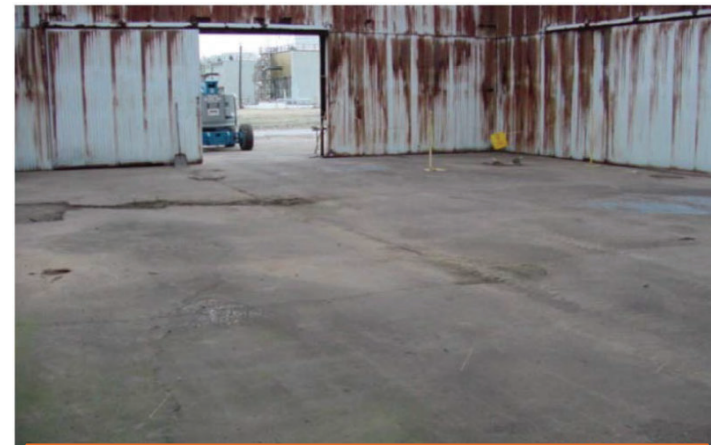
Interior view after completion of the DMSA removal
