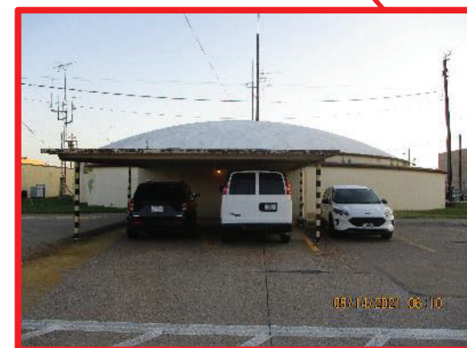
C-300 Building Photo: 9/2021
