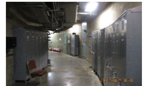
Basement Hallway looking East
