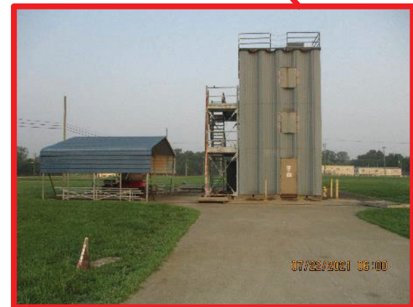
C-207 Fire Training Facility Photo: 7/2021 2
