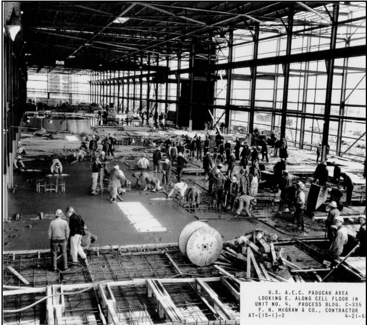
Fig. 11. Construction work on the interior of Building C-335 in April 1952.
