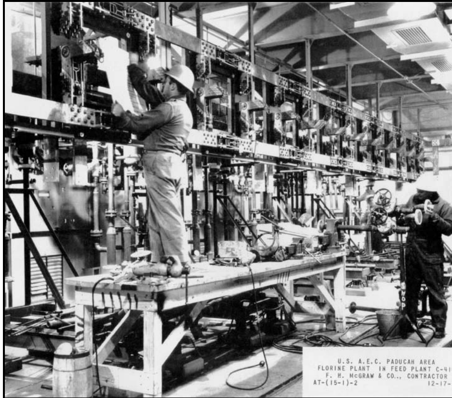
Fig. 12. Construction of the fluorine cell room electrical buss work in the C-410 Complex in December 1952.
