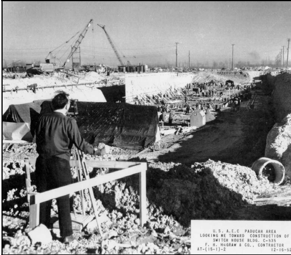
Fig. 10. Construction activity at the plant in December 1952.
