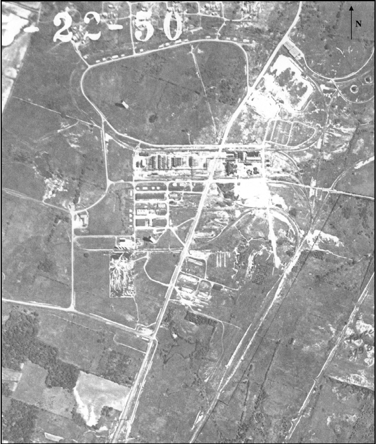
Fig. 5. Aerial view of the KOW TNT Production Area in May 1950. (Photograph on file at the McCracken County Property Valuation Office, Paducah, Kentucky.)
