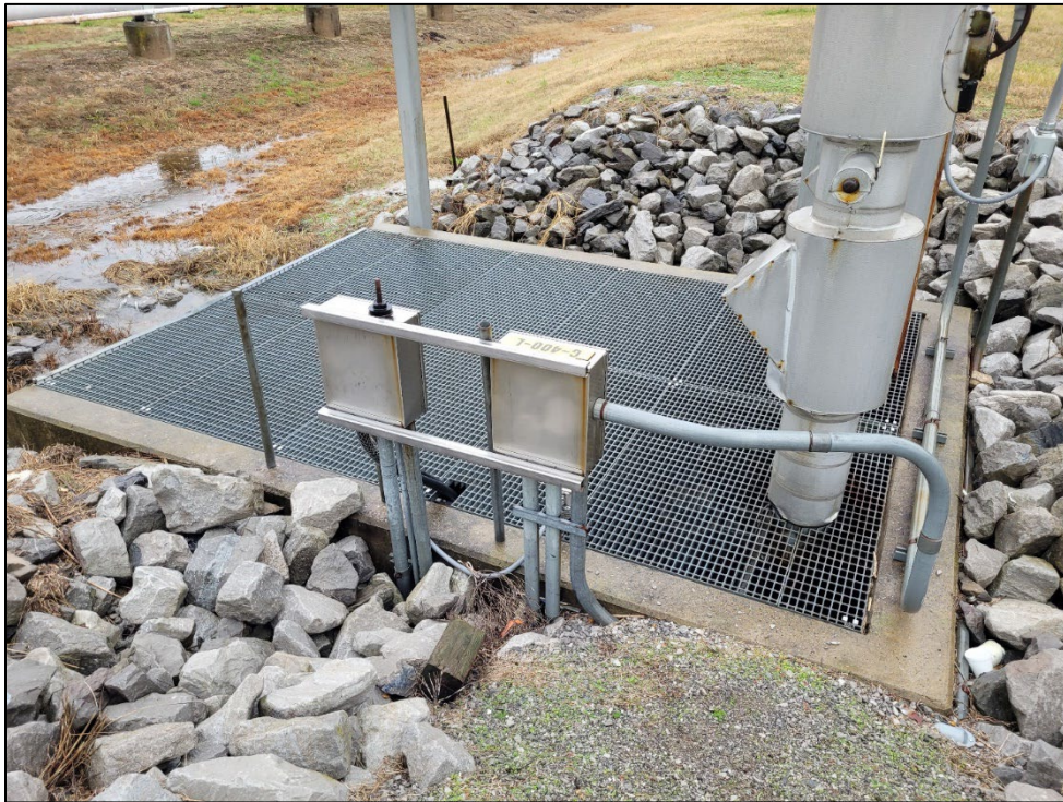
Figure 11.2. C-400-L Lift Station
