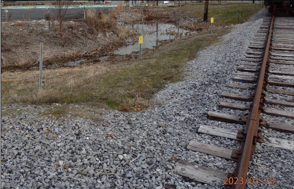
Figure 16.2. KPDES Outfall 001 Internal Ditches, January 18, 2023 (Looking Northwest)
