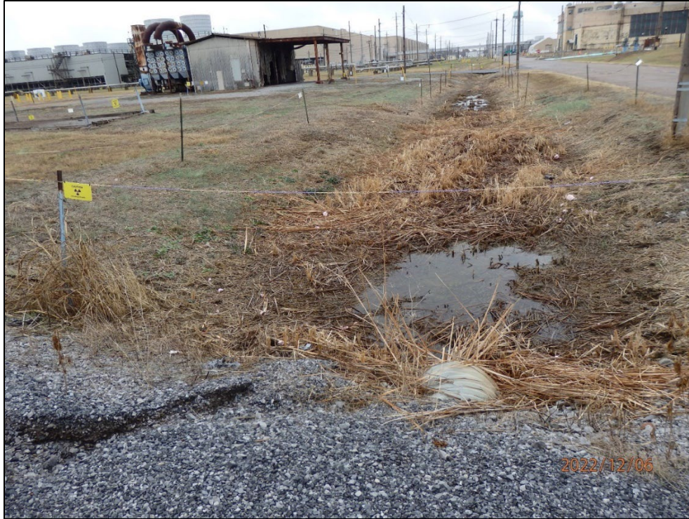
Figure 16.4. KPDES Outfall 015 Internal Ditches, December 6, 2022 (Looking East)
