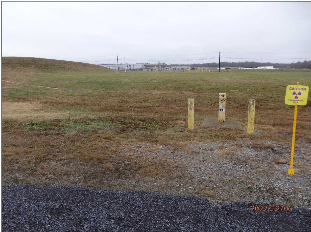
Figure 17.2. C-749 Uranium Burial Ground (Looking South)
