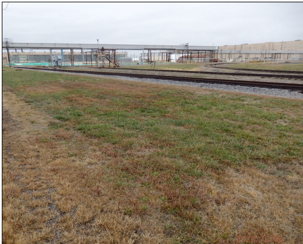
Figure 16.3. KPDES Outfall 010 Internal Ditch and Area, December 6, 2022 (Looking West)
