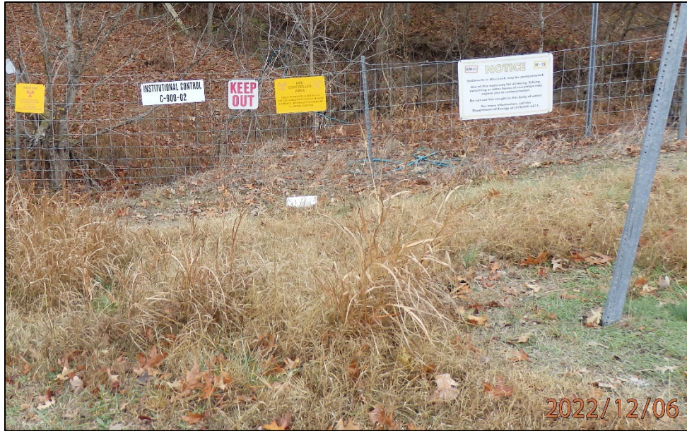
Figure 15.4. Sign and Fencing Installed for the Surface Water ICM
