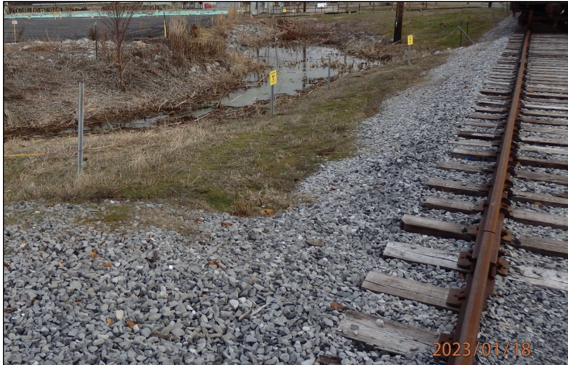
Figure 16.2. KPDES Outfall 001 Internal Ditches, January 18, 2023 (Looking Northwest)
