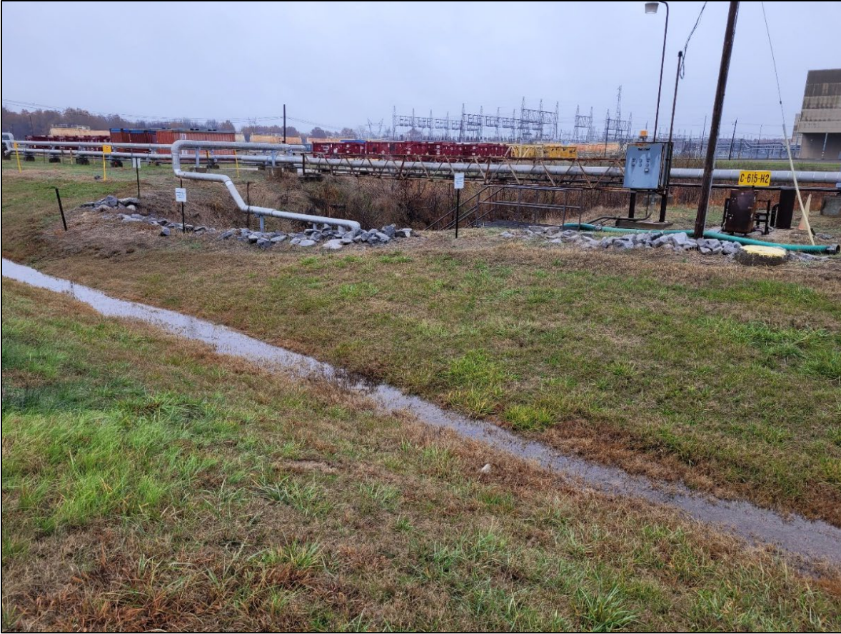
Figure 12.3. NSDD and Gabion Structure
