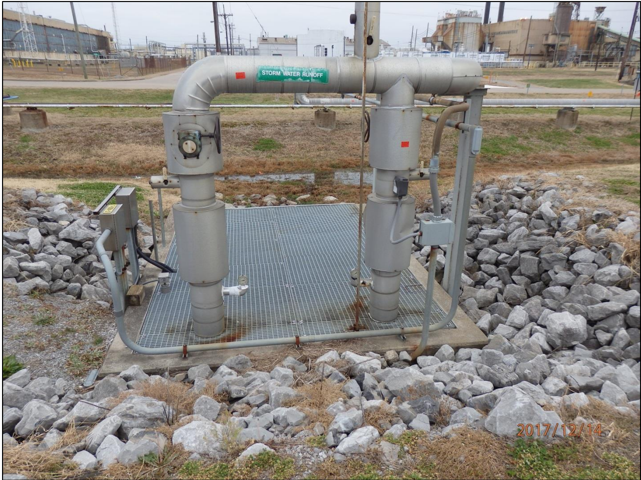
Figure 11.2. C-400-L Lift Station
