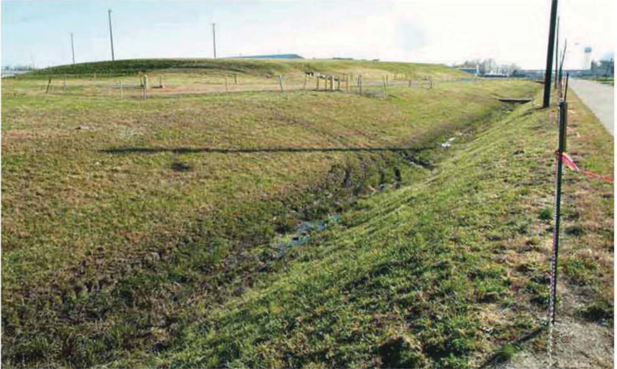
Figure 16.12. Outfall 015 EU03 11-12-09 (Before)
