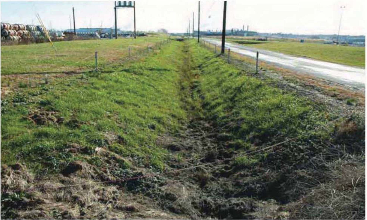
Figure 16.11. Outfall 015, EU02 11-12-09 (Before)
