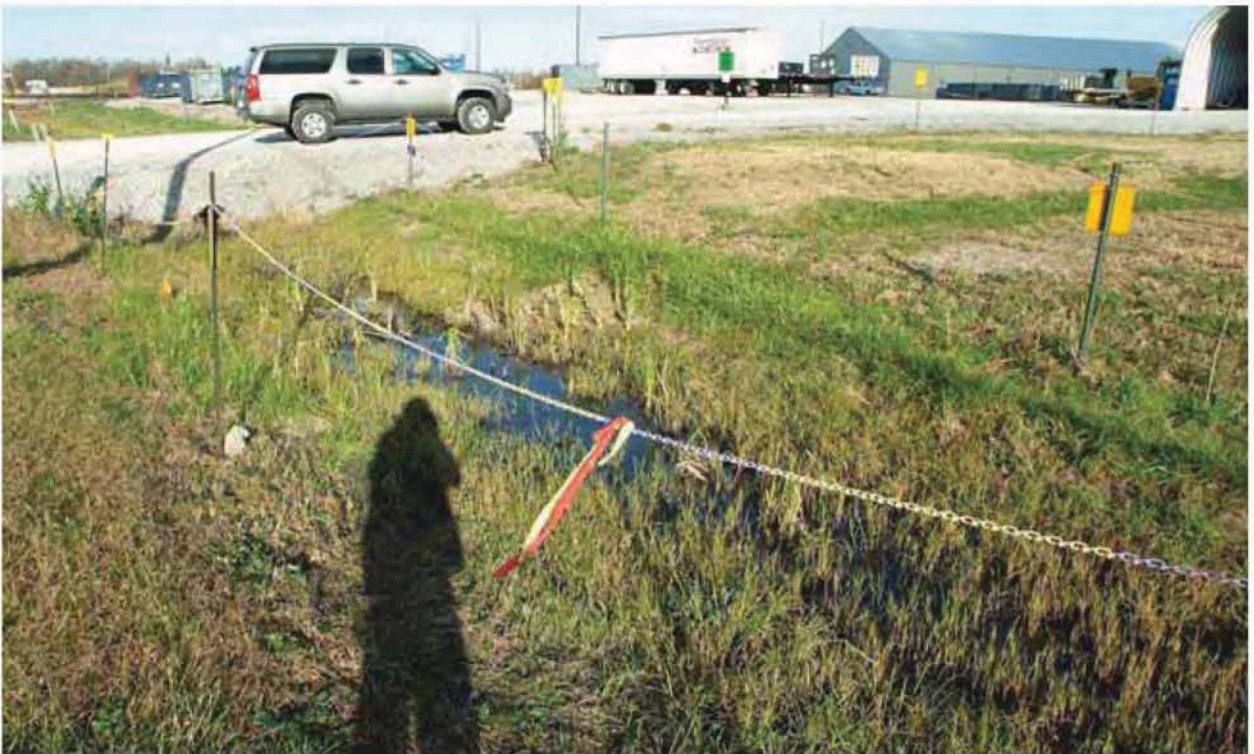
Figure 16.15. Outfall 015 EU04 11-12-09 (Before)
