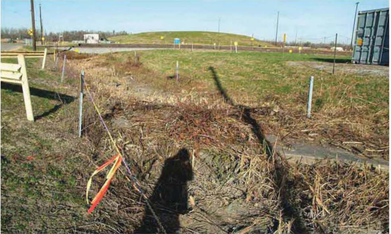
Figure 16.16. Outfall 015 EU04 11-12-09 (Before)
