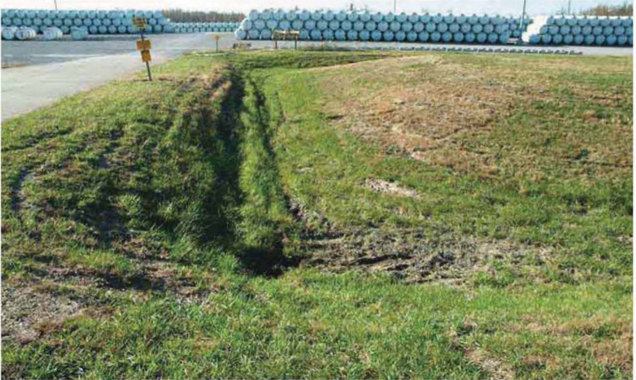
Figure 16.18. Outfall 015 EU08 11-12-09 (Before)
