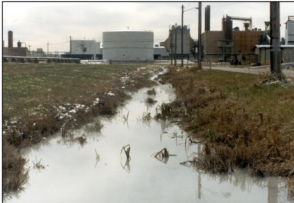
Figure 12.2. NSDD Sections 1 and 2 before Remedial Action
