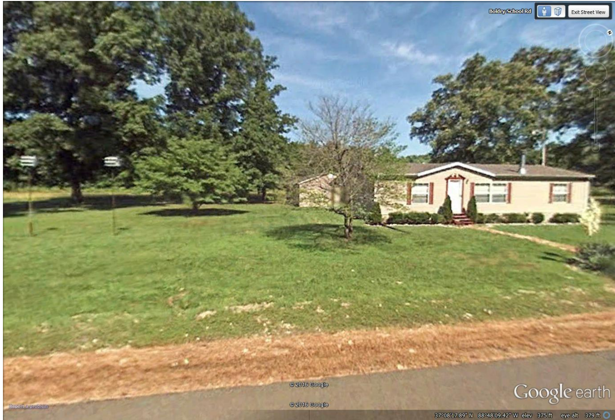
Figure 6. Property 2 Street View—Residence
