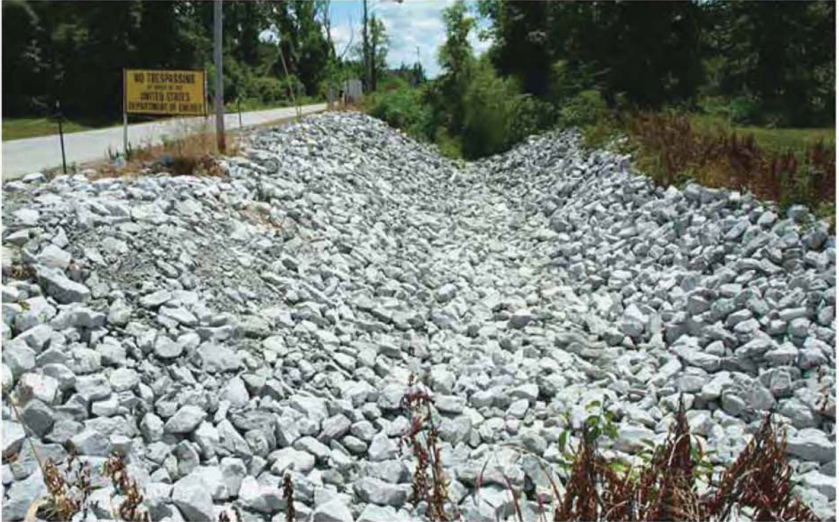
Figure 16.32. North South Diversion Ditch Section 3 EU 03 07-13-10 (After)
