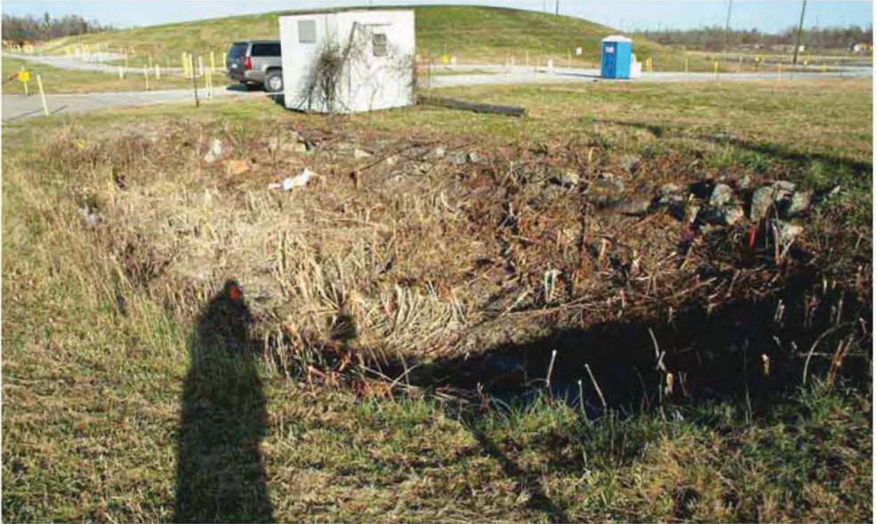
Figure 16.14. Outfall 015 EU04 11-12-09 (Before)
