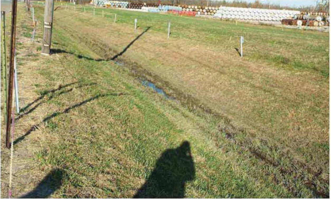
Figure 16.10. Outfall 015, EU02 11-12-09 (Before)
