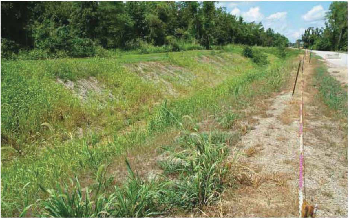
Figure 16.31. North South Diversion Ditch Section 3 EU 02 07-13-10 (After)
