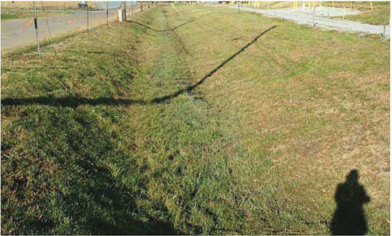
Figure 16.13. Outfall 015 EU03 11-12-09 (Before)
