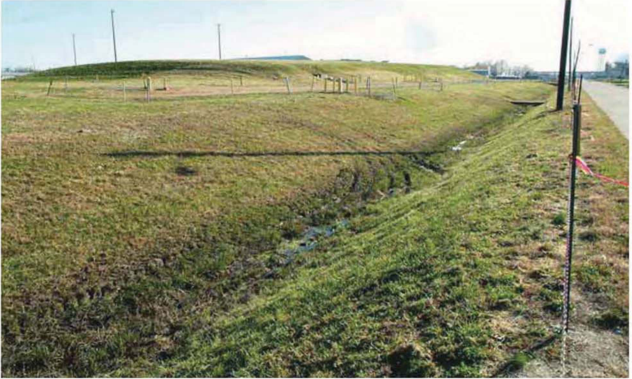
Figure 16.12. Outfall 015 EU03 11-12-09 (Before)
