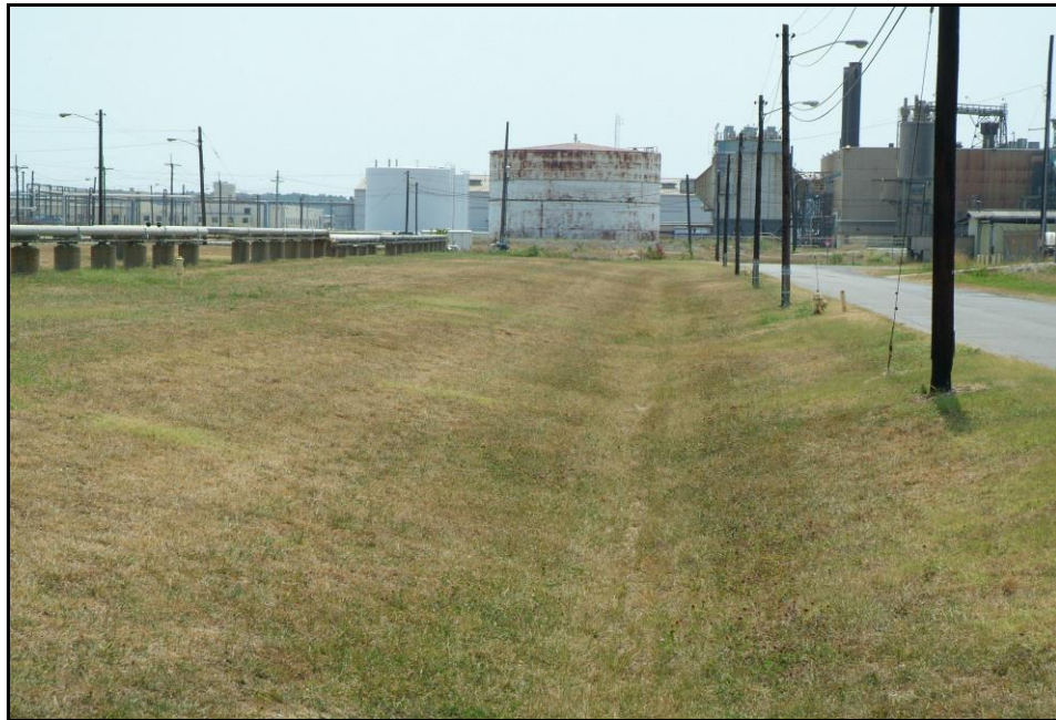
Figure 12.3. NSDD Sections 1 and 2 after Remedial Action
