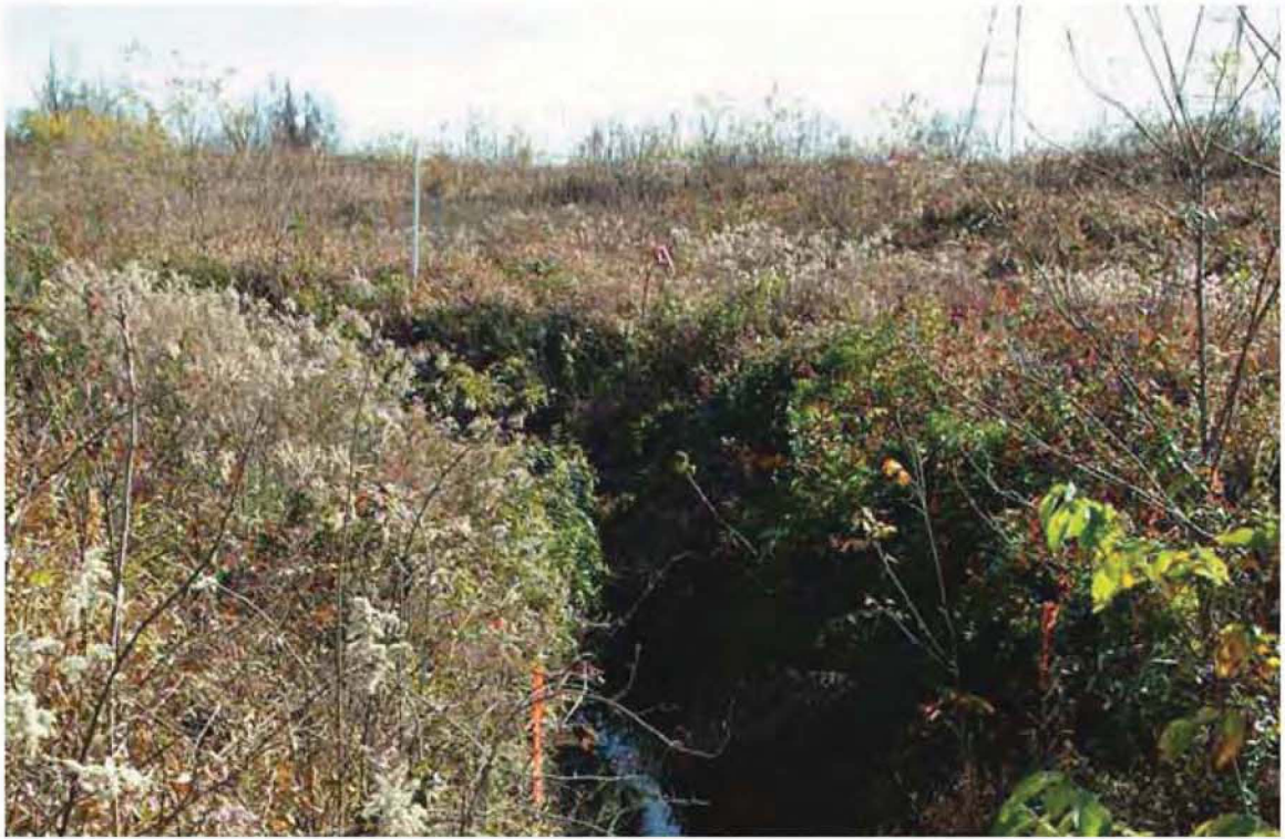
Figure 16.29. North South Diversion Ditch Section 5 11-12-09 (Before)
