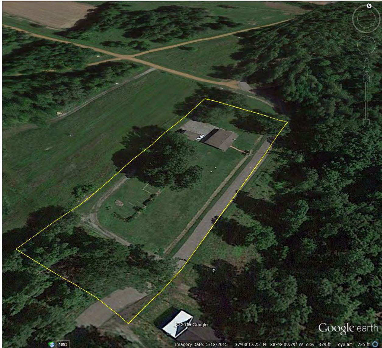
Property 2 Aerial View
