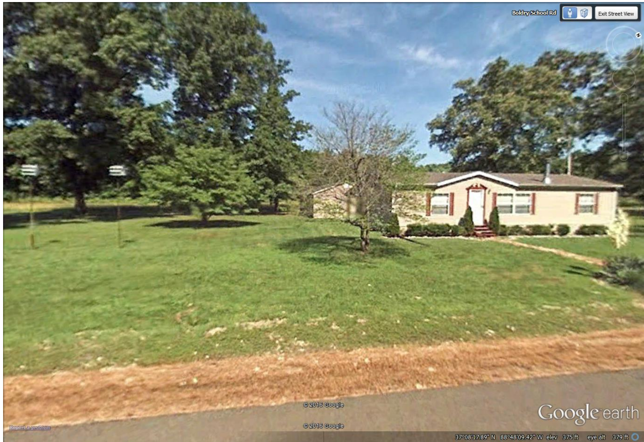
Figure 6. Property 2 Street View—Residence
