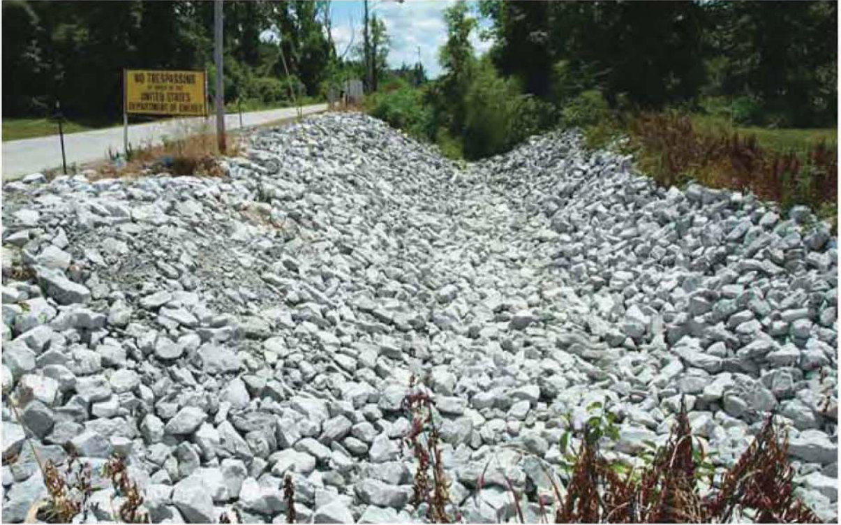
Figure 16.32. North South Diversion Ditch Section 3 EU 03 07-13-10 (After)
