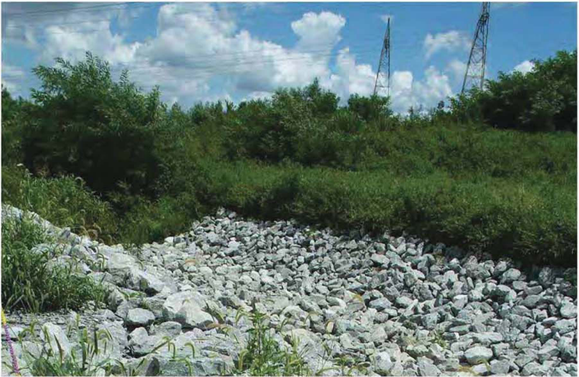
Figure 16.33. North South Diversion Ditch Section 5 07-13-10 (After)
