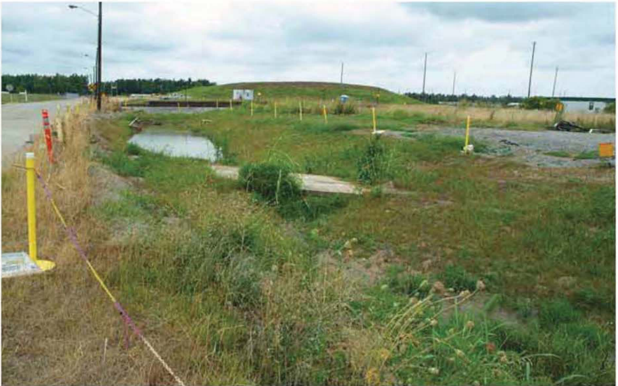
Figure 16.22. Outfall 015, Eu 04 07-12-10 (After)
