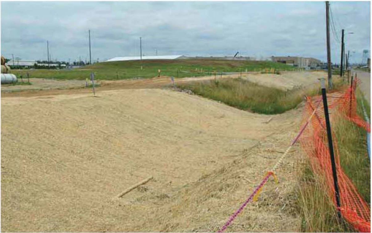
Figure 16.20. Outfall 015, EU 02/03 07-12-10 (After)
