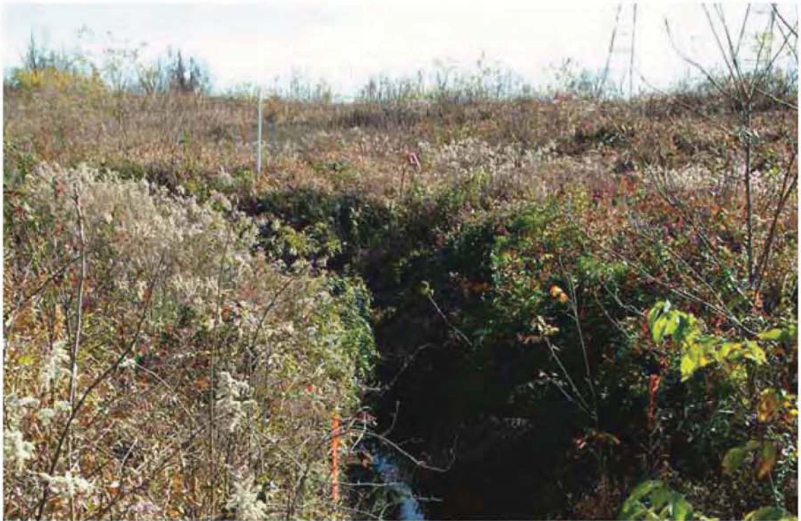
Figure 16.29. North South Diversion Ditch Section 5 11-12-09 (Before)
