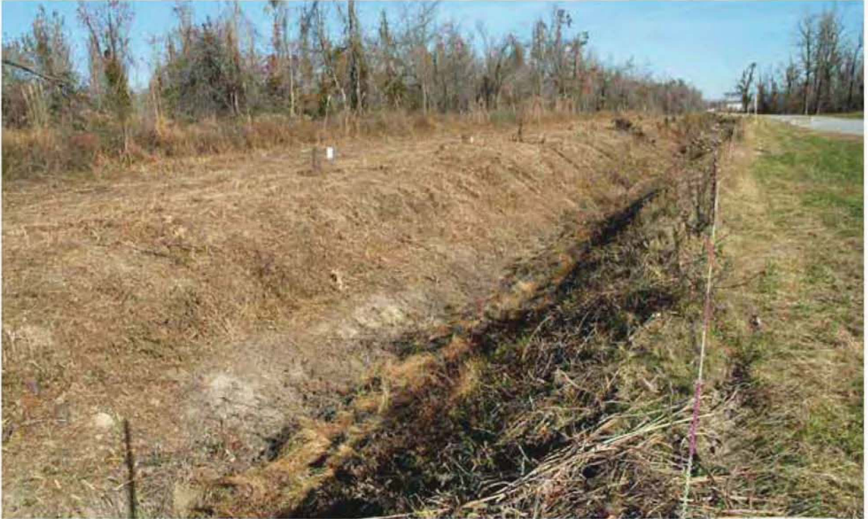
Figure 16.25. North South Diversion Ditch Section 3, EU 02 11-12-09 (Before)
