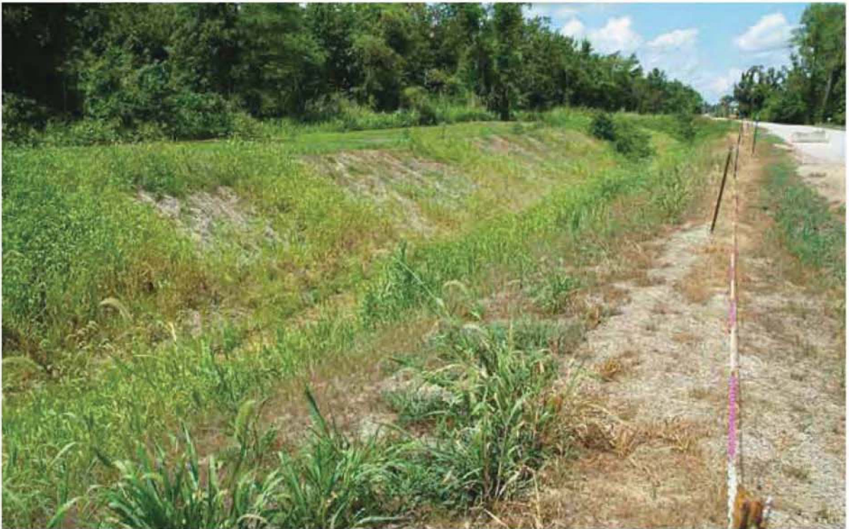
Figure 16.31. North South Diversion Ditch Section 3 EU 02 07-13-10 (After)
