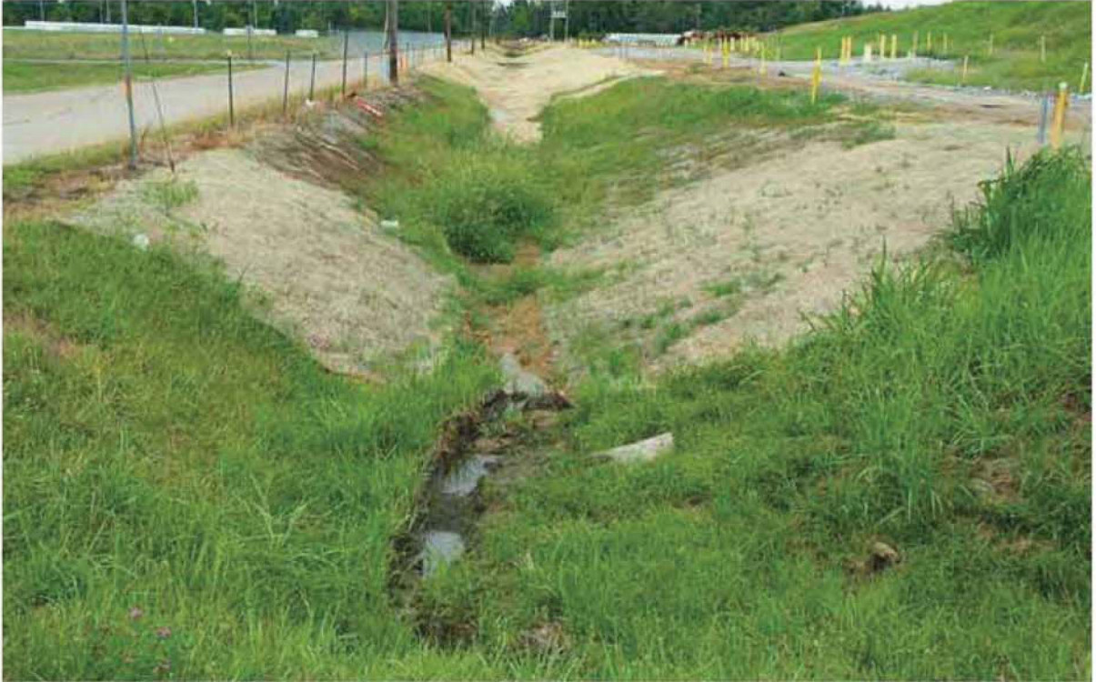
Figure 16.21. Outfall 015, EU 03 07-12-10 (After)
