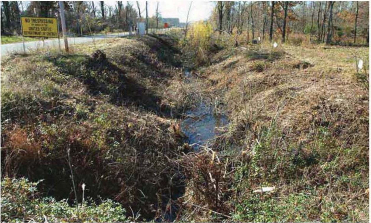
Figure 16.26. North South Diversion Ditch Section 3, EU 03 11-12-09 (Before)
