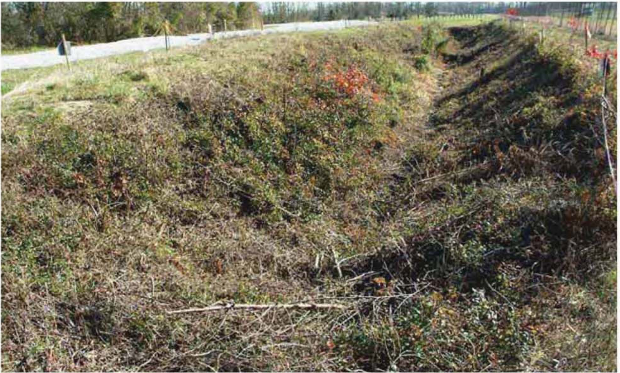
Figure 16.24. North South Diversion Ditch Section 3, E U01 11-12-09 (Before)
