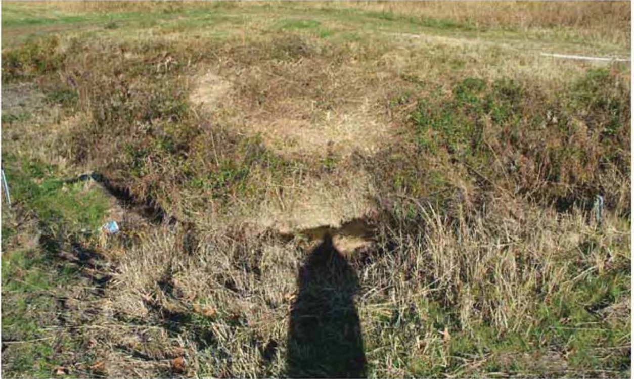
Figure 16.27. North South Diversion Ditch Section 3, EU 03 11-12-09 (Before)
