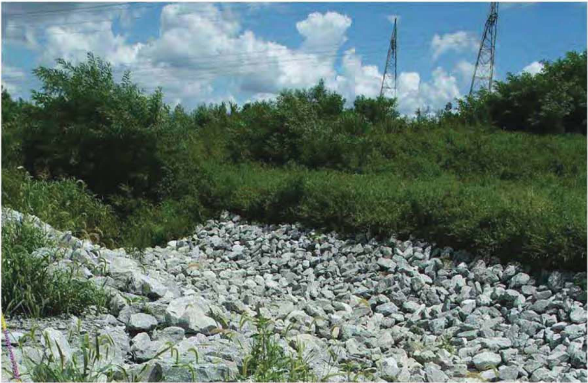
Figure 16.33. North South Diversion Ditch Section 5 07-13-10 (After)
