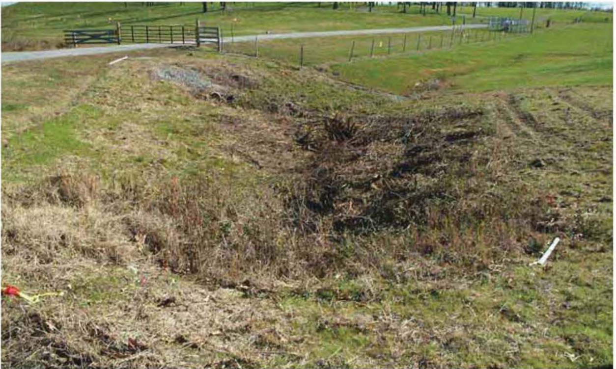
Figure 16.28. North South Diversion Ditch Section 3, EU 03 11-12-09 (Before)
