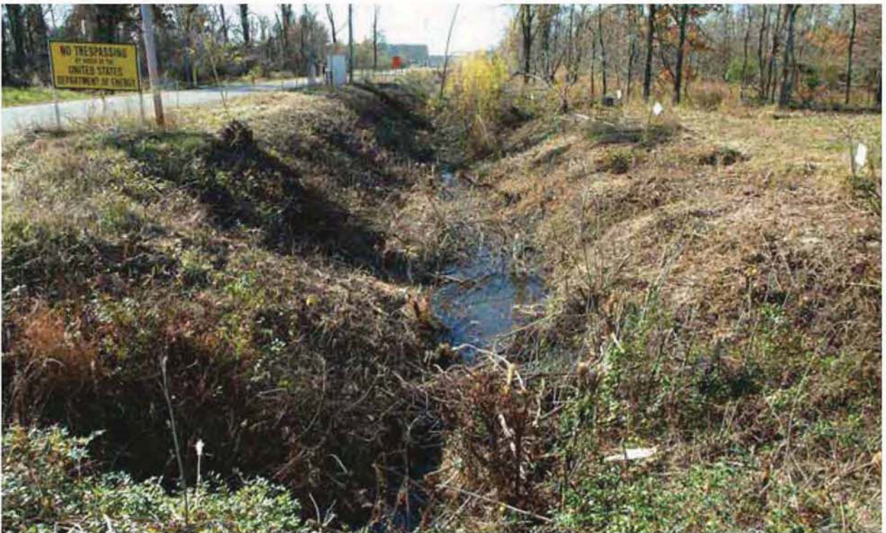
Figure 16.26. North South Diversion Ditch Section 3, EU 03 11-12-09 (Before)
