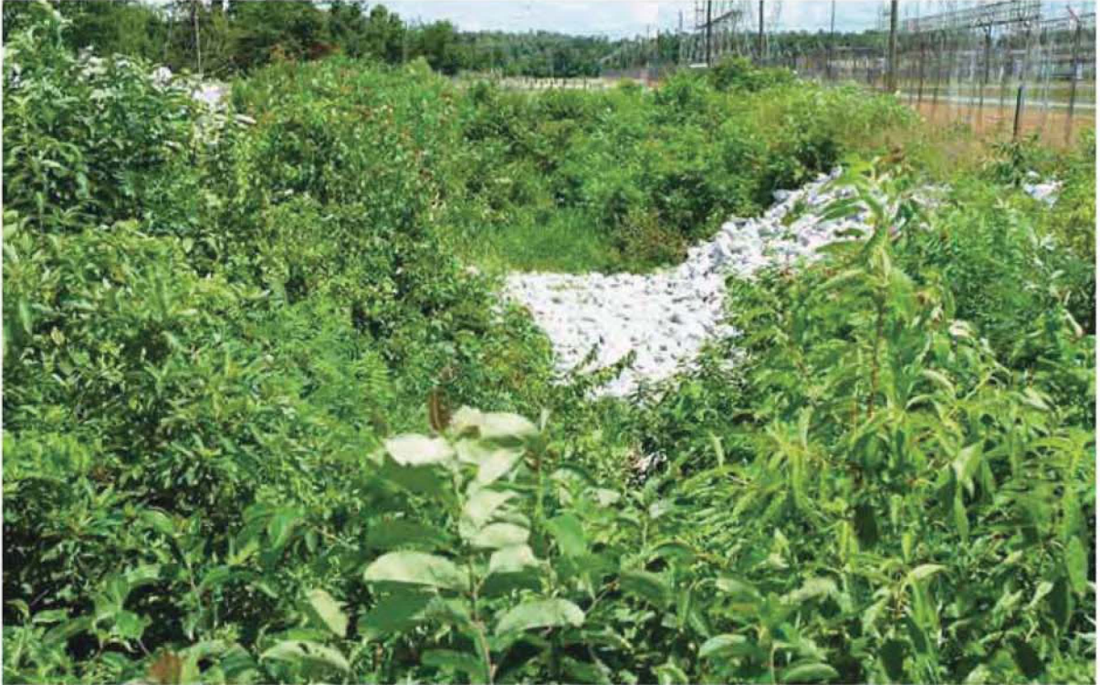
Figure 16.30. North South Diversion Ditch Section 3 EU 01 07-13-10 (After)
