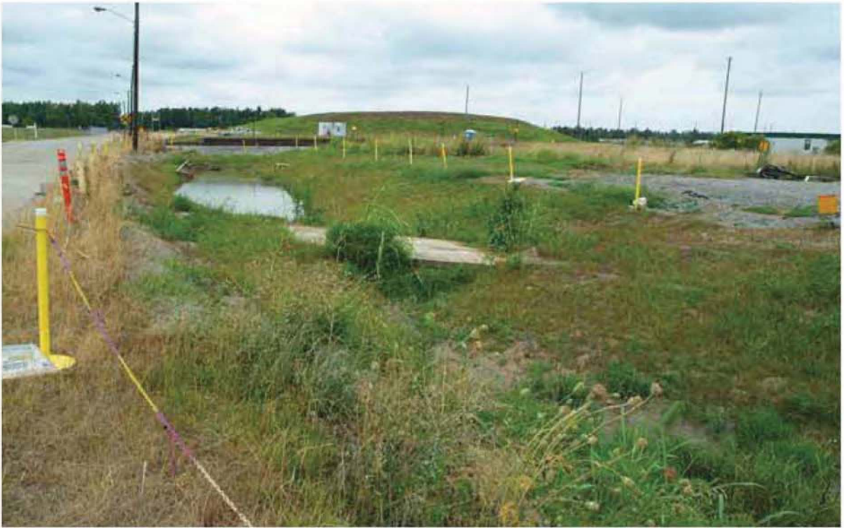
Figure 16.22. Outfall 015, Eu 04 07-12-10 (After)
