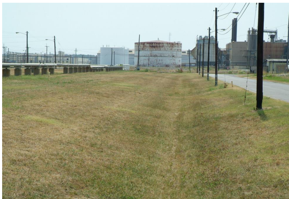
Figure 12.3. NSDD Sections 1 and 2 After Remedial Action
