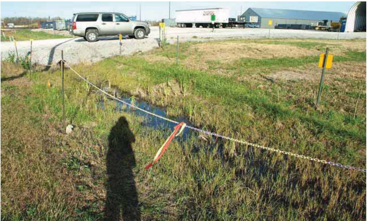
Figure 16.15. Outfall 015 EU04 11-12-09 (Before)
