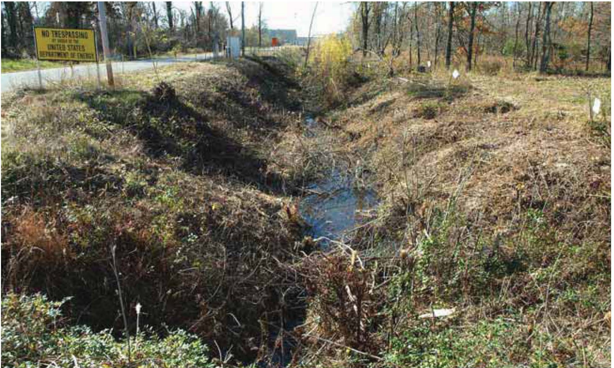
Figure 16.26. North South Diversion Ditch Section 3, EU 03 11-12-09 (Before)
