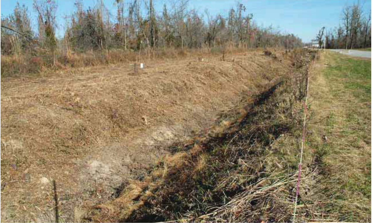
Figure 16.25. North South Diversion Ditch Section 3, EU 02 11-12-09 (Before)
