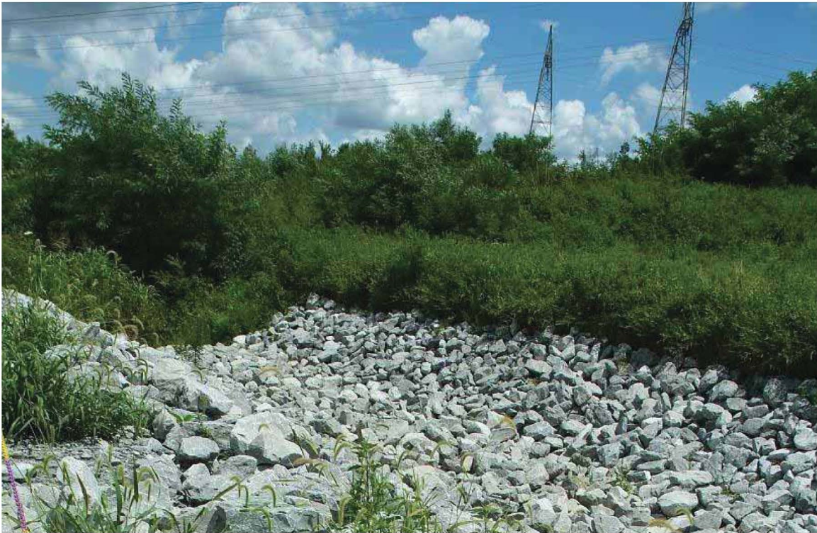
Figure 16.33. North South Diversion Ditch Section 5 07-13-10 (After)
