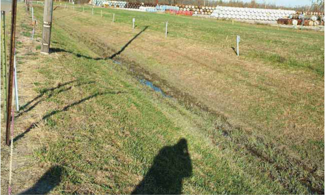
Figure 16.10. Outfall 015, EU02 11-12-09 (Before)
