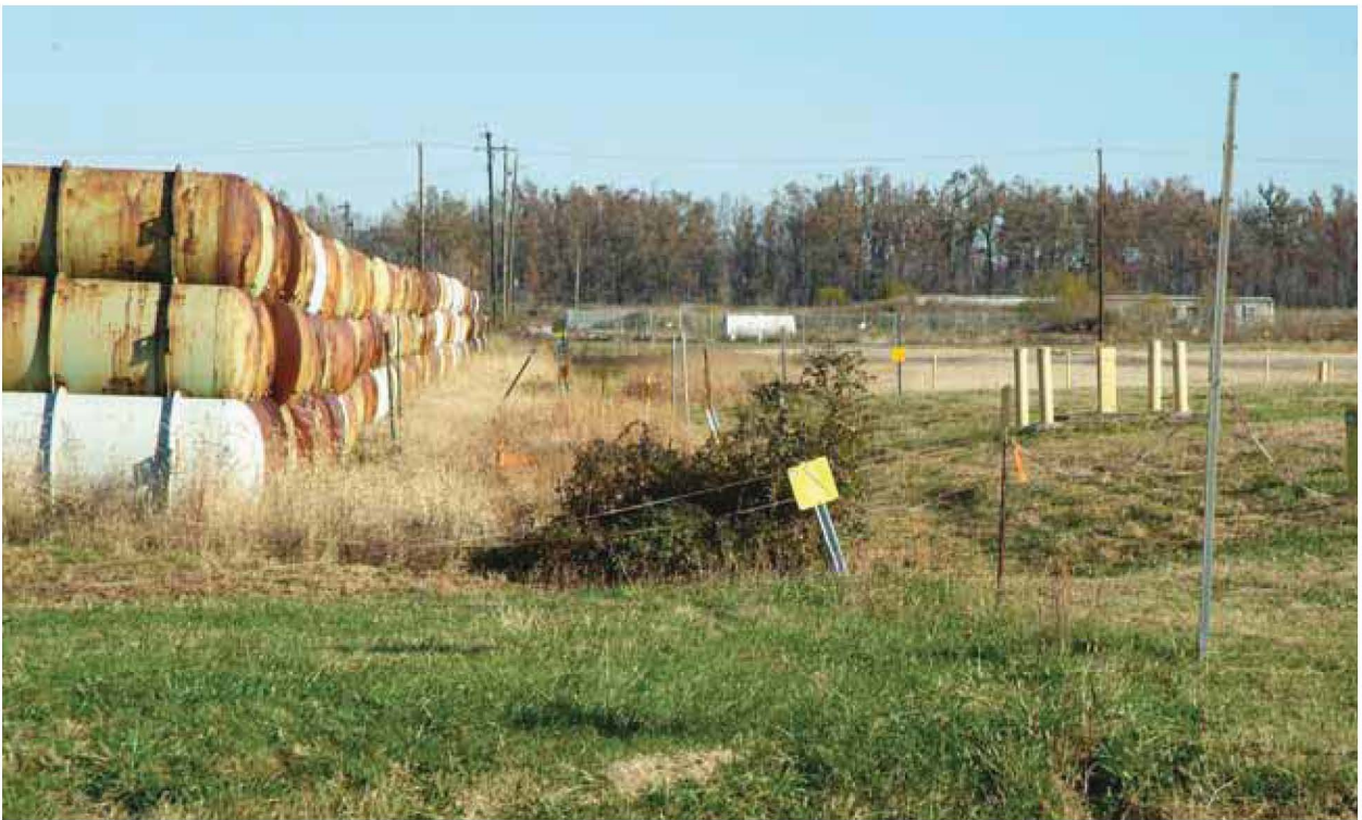
Figure 16.17. Outfall 015 EU07 11-12-09 (Before)
