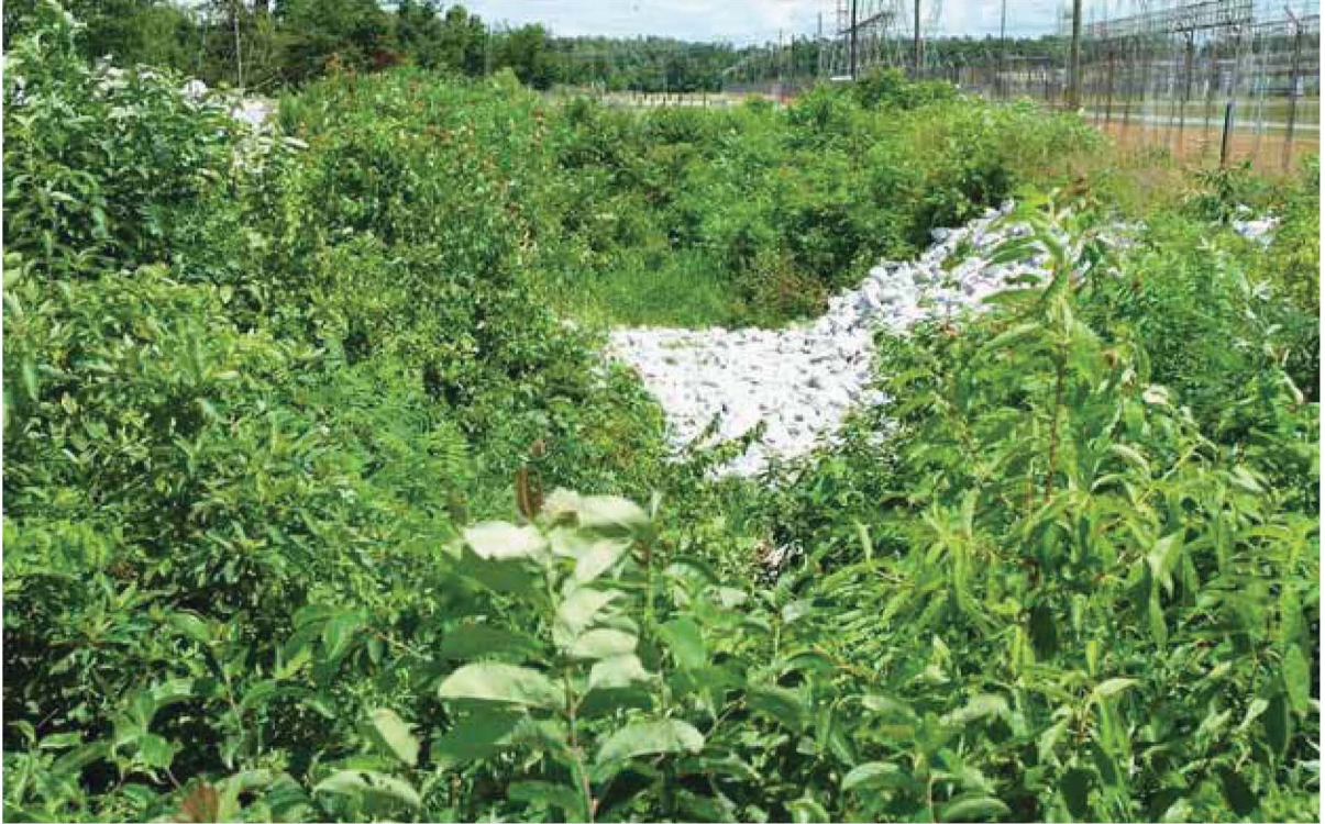
Figure 16.30. North South Diversion Ditch Section 3 EU 01 07-13-10 (After)
