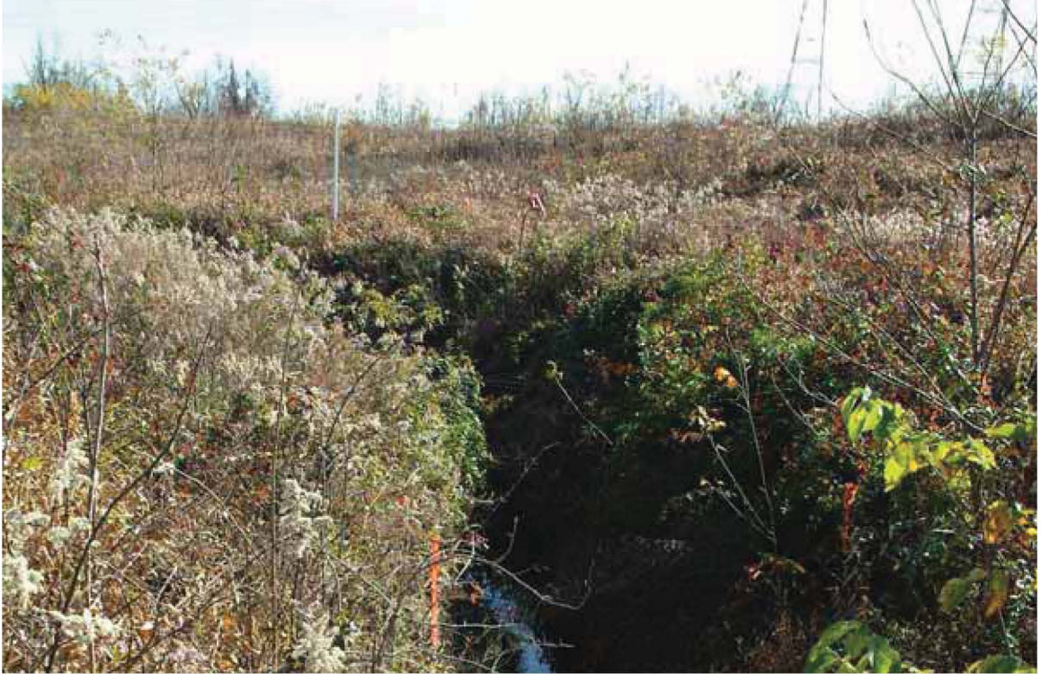
Figure 16.29. North South Diversion Ditch Section 5 11-12-09 (Before)
