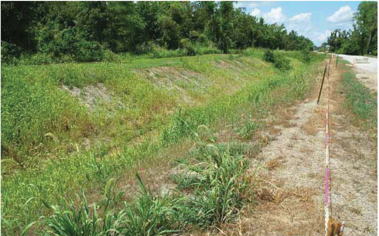
Figure 16.31. North South Diversion Ditch Section 3 EU 02 07-13-10 (After)
