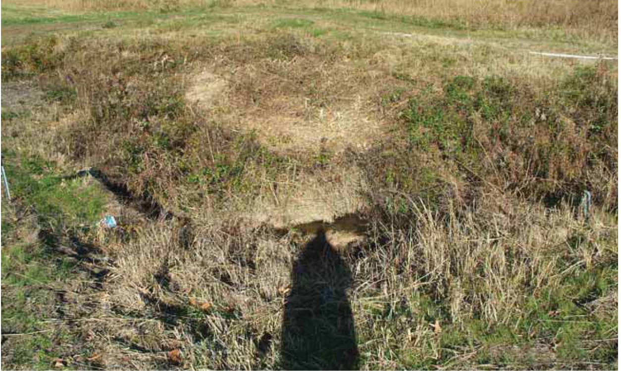
Figure 16.27. North South Diversion Ditch Section 3, EU 03 11-12-09 (Before)
