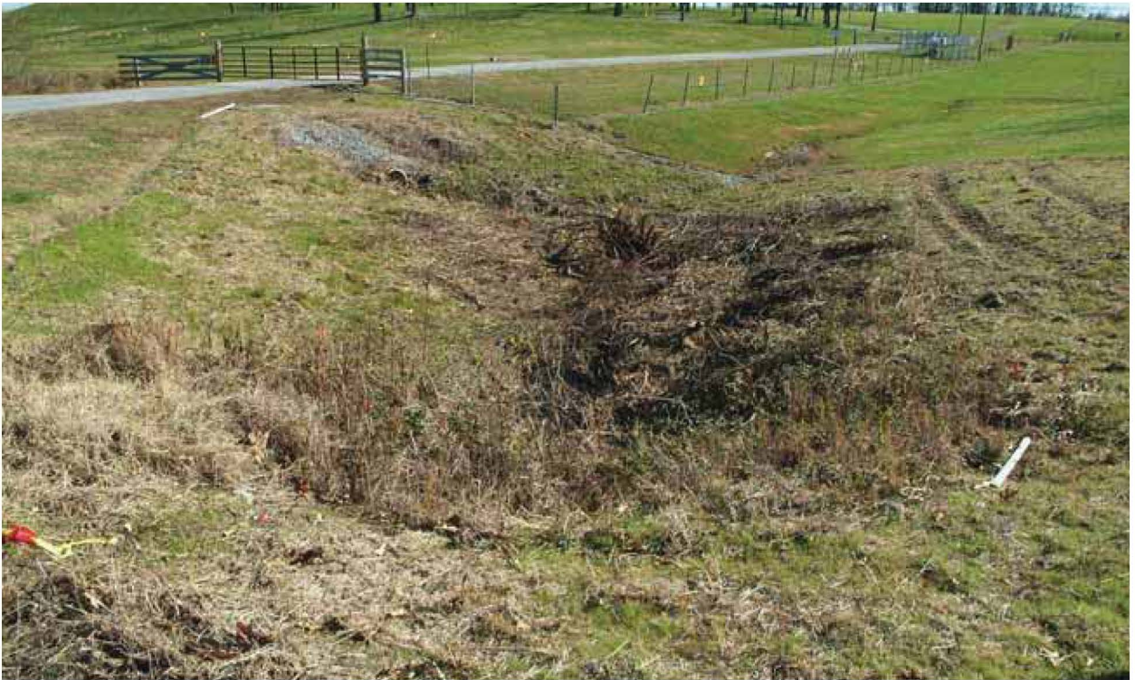
Figure 16.28. North South Diversion Ditch Section 3, EU 03 11-12-09 (Before)
