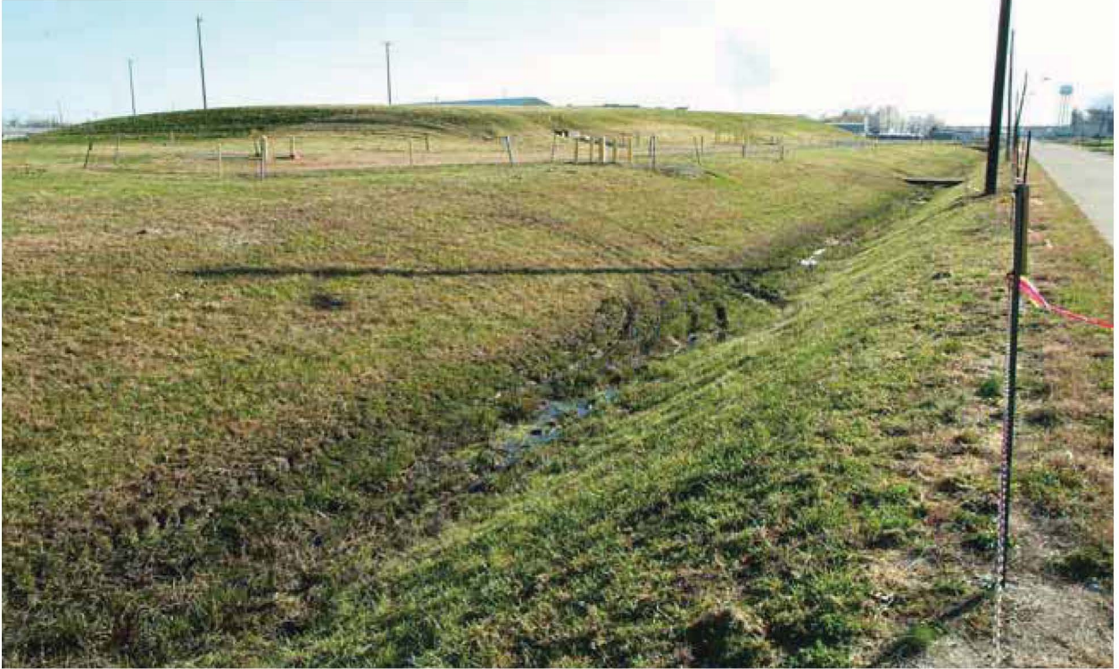
Figure 16.12. Outfall 015 EU03 11-12-09 (Before)
