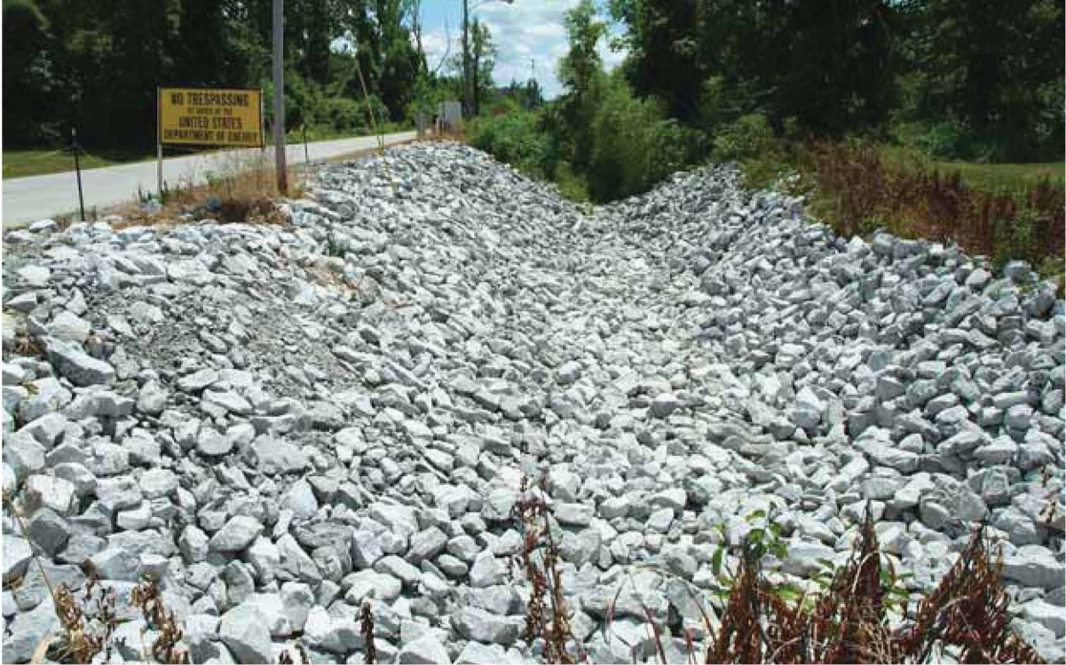
Figure 16.32. North South Diversion Ditch Section 3 EU 03 07-13-10 (After)
