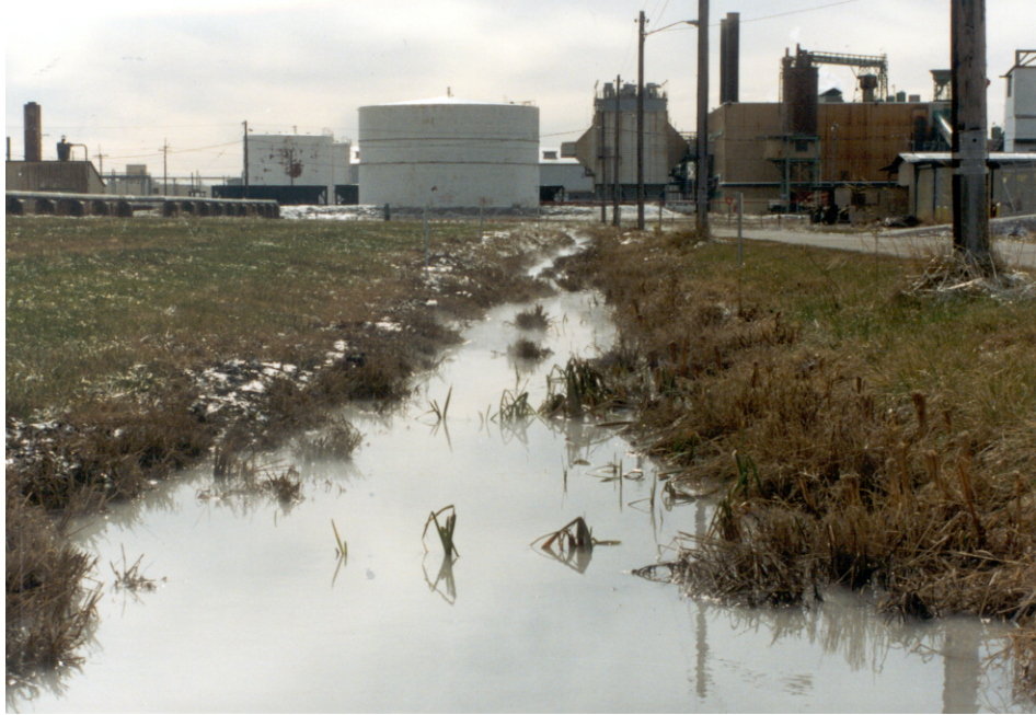
Figure 10.1. NSDD Sections 1 and 2 Before Remedial Action
