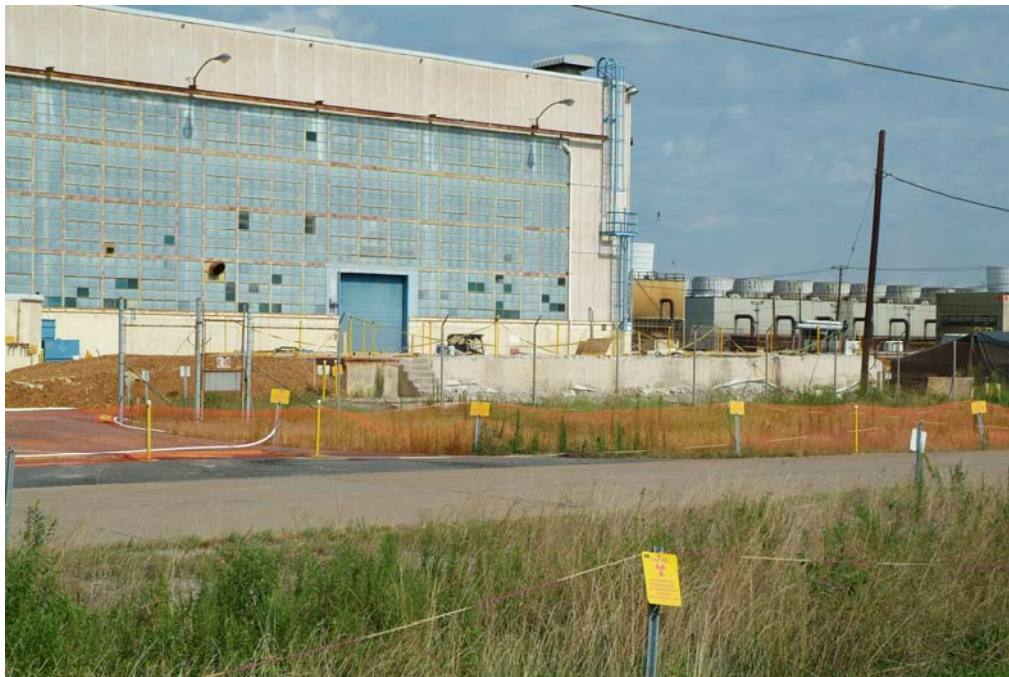
Figure 15.2. C-402 Lime House After D&D
