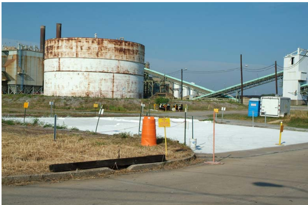
Figure 16.2. C-405 After Demolition
