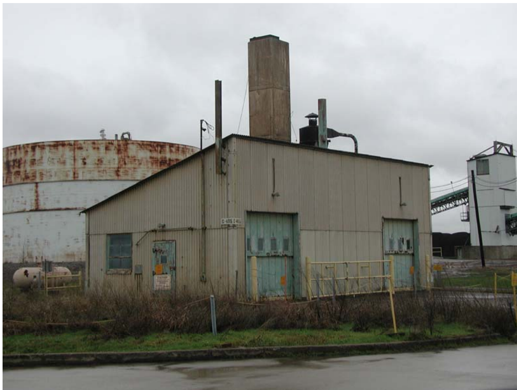
Figure 16.1. C-405 Incinerator Before Demolition
