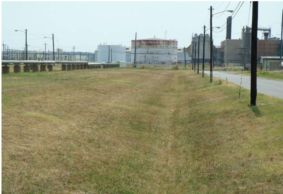
Figure 10.2. NSDD Sections 1 and 2 After Remedial Action
