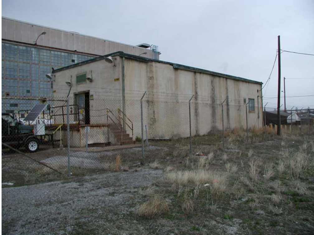
Figure 15.1. C-402 Lime House Before D&D
