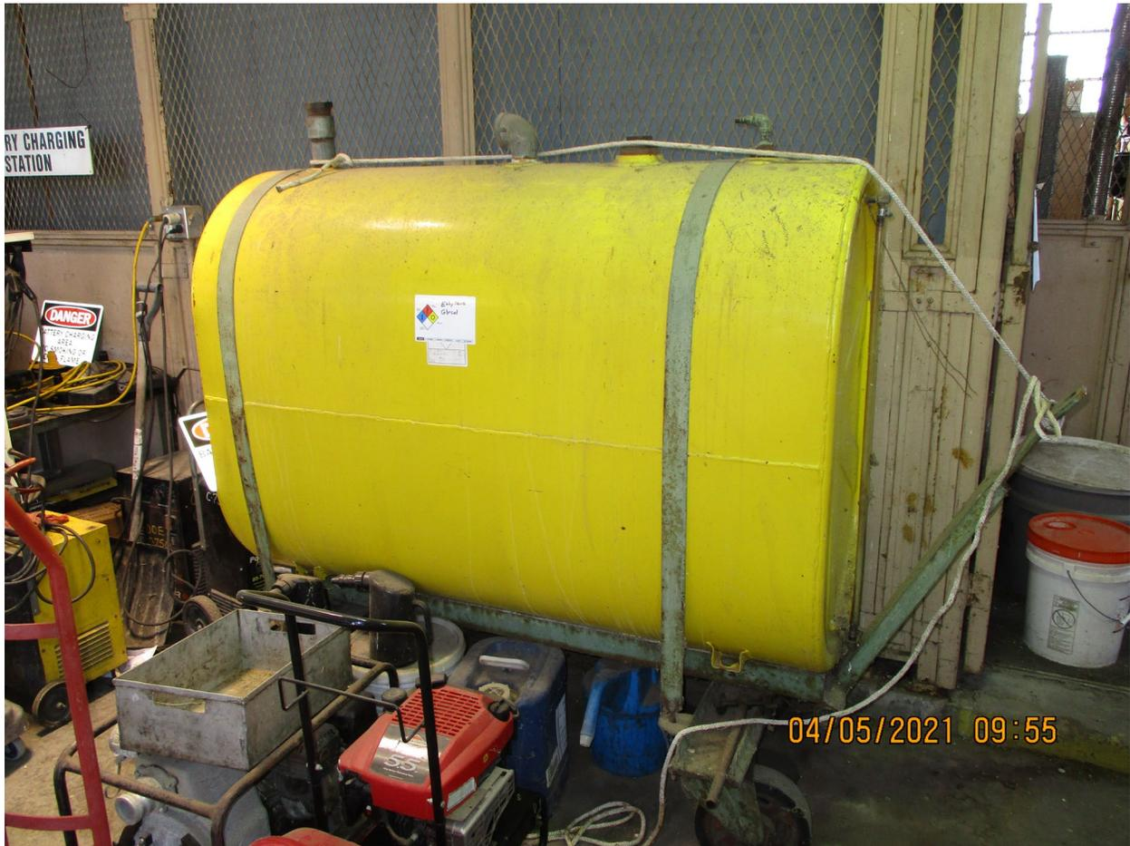
Figure 11. Ethylene Glycol Storage Tank
