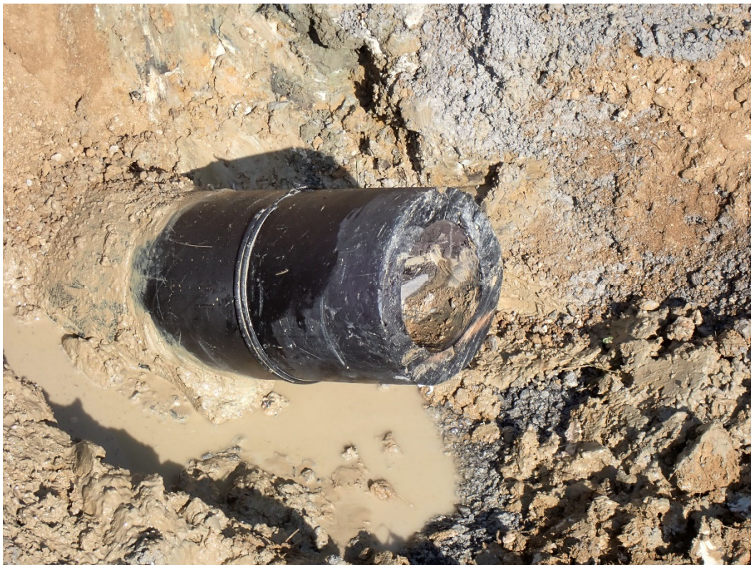
Photo 2, HDPE Stub to be capped
