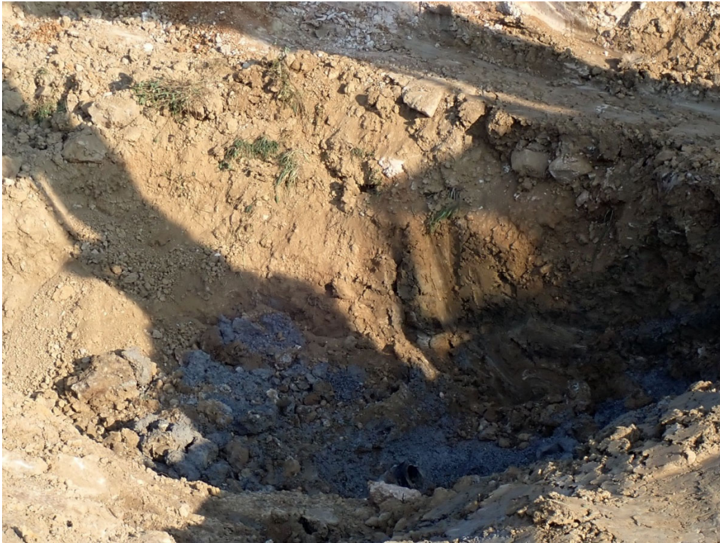
Photo 1, Excavation exposing the Y-fitting
