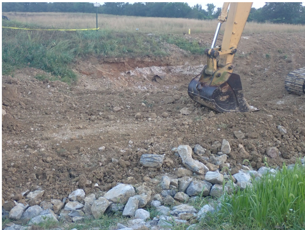
Photo 6, Backfilling the excavation
