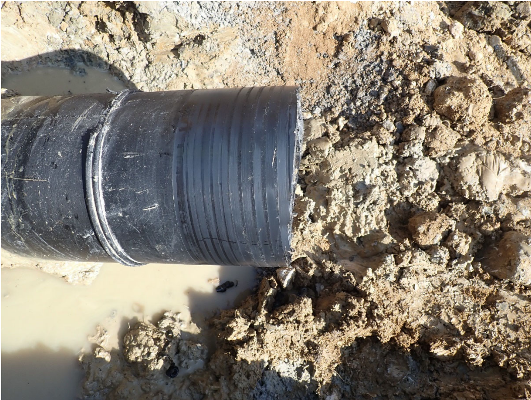
Photo 3, HDPE Stub prepared to receive cap
