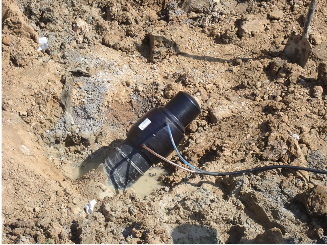
Photo 4, HDPE Electrofusion Cap being installed
