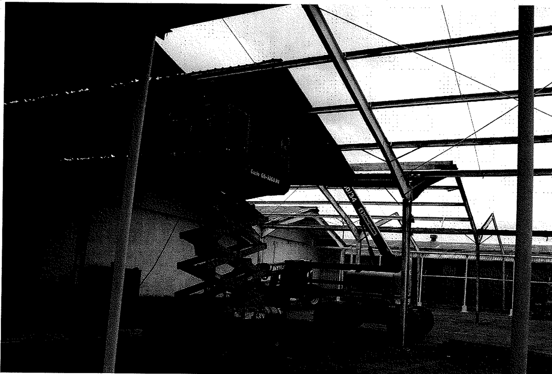
Figure 7. Photograph of Structure Removal of C-746-A West End Smelter
