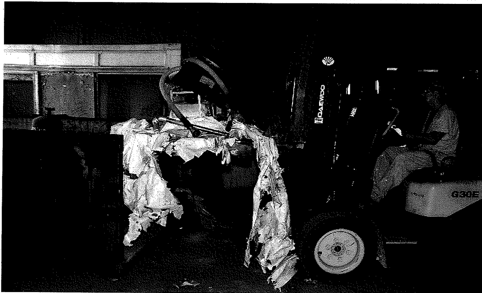
Figure 6. Photograph of Loose Material Removal at C-746-A West End Smelter
