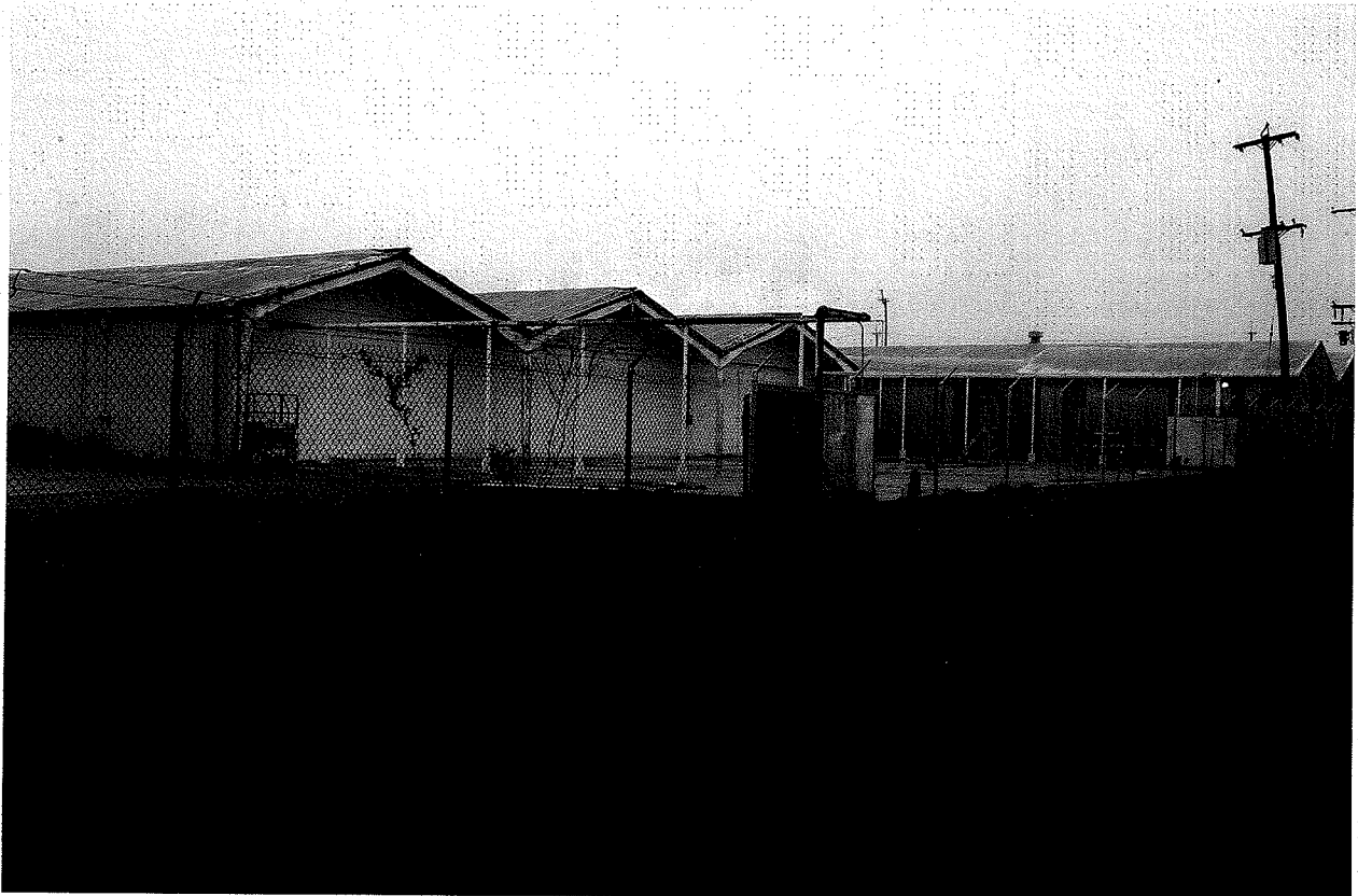
Figure 8. Photograph of C-746-A West End Smelter Post D&D
