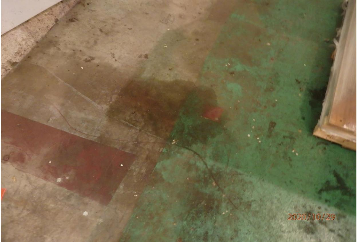
**Figure 12. Floor Stains Across from and Outside of the Footprint of the Spray Paint Booth**
