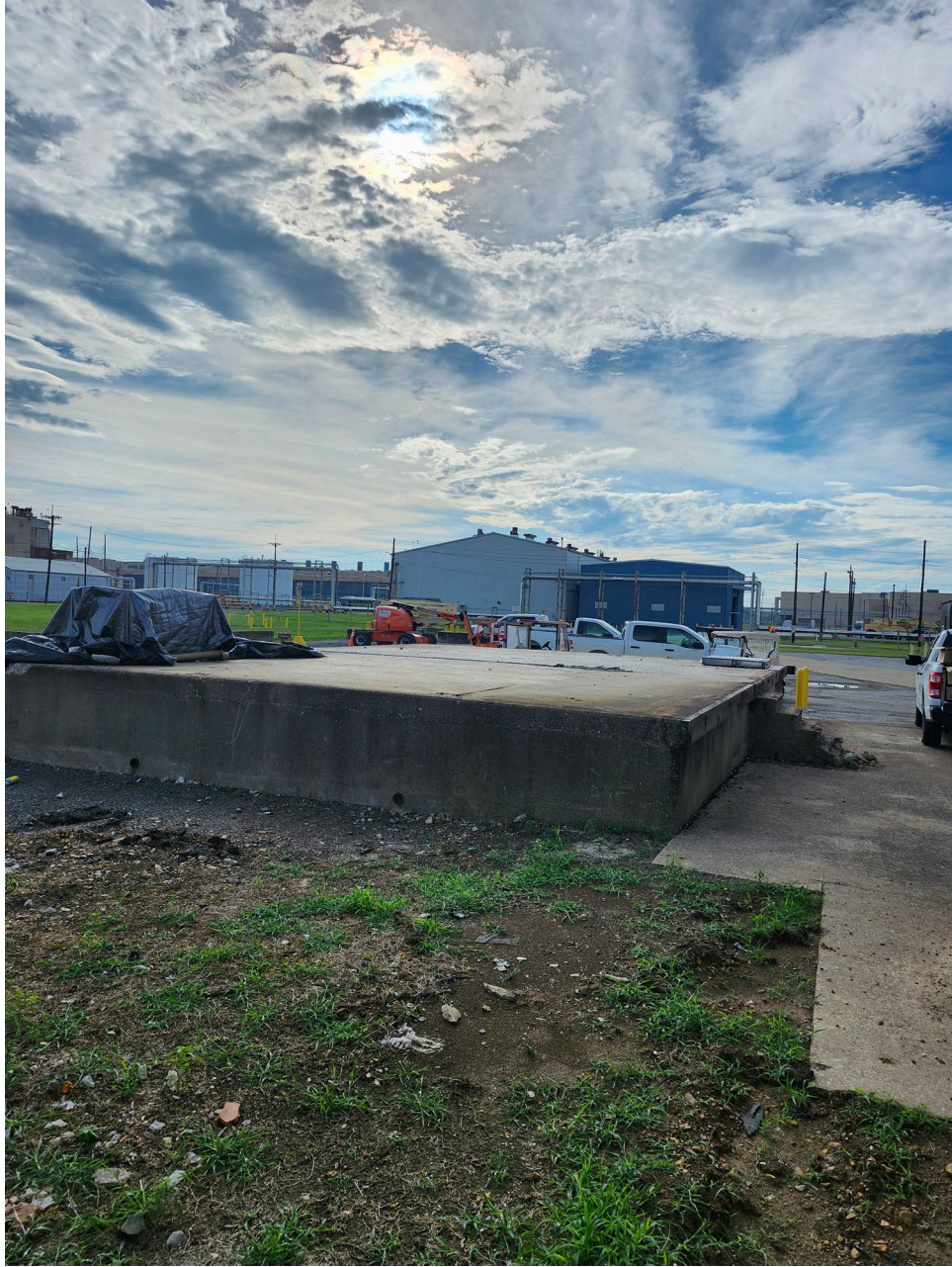
Figure 5. Remaining C-721 Slab Facing East (June 2024)
