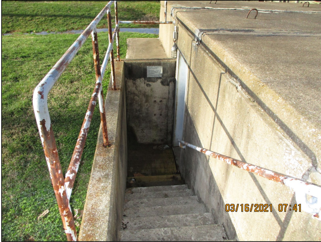
Figure 6. Stairs Leading to the Booster Pump Station Plant Water Entrance
