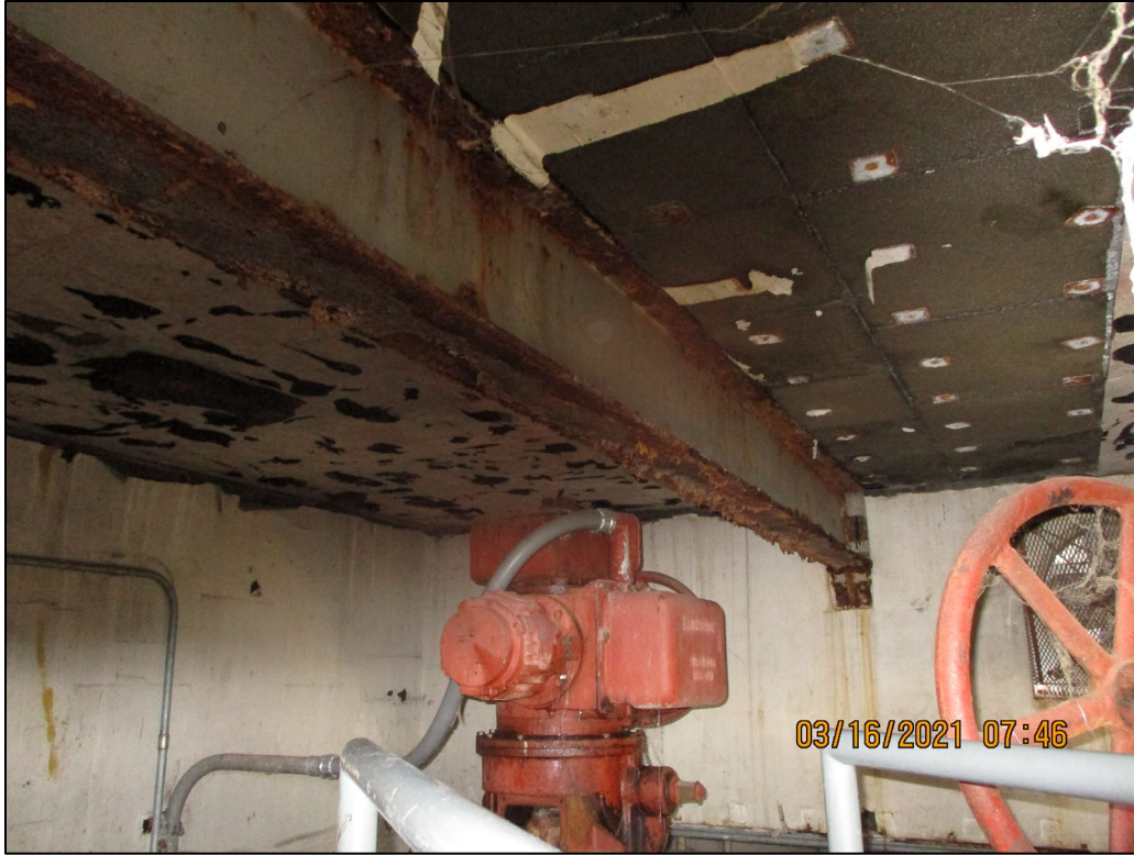
Figure 8. Interior View of the Ceiling in the Southwest Corner
