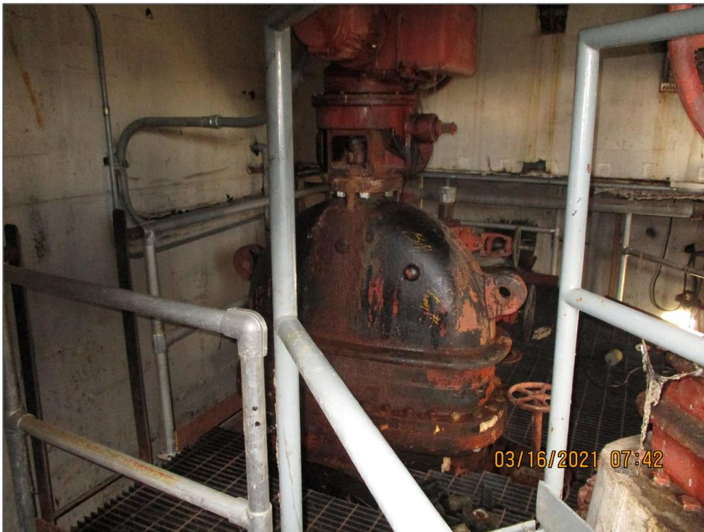
**Figure 7. Interior View of C-611-T Showing the Plant Water Inlet Valve**
