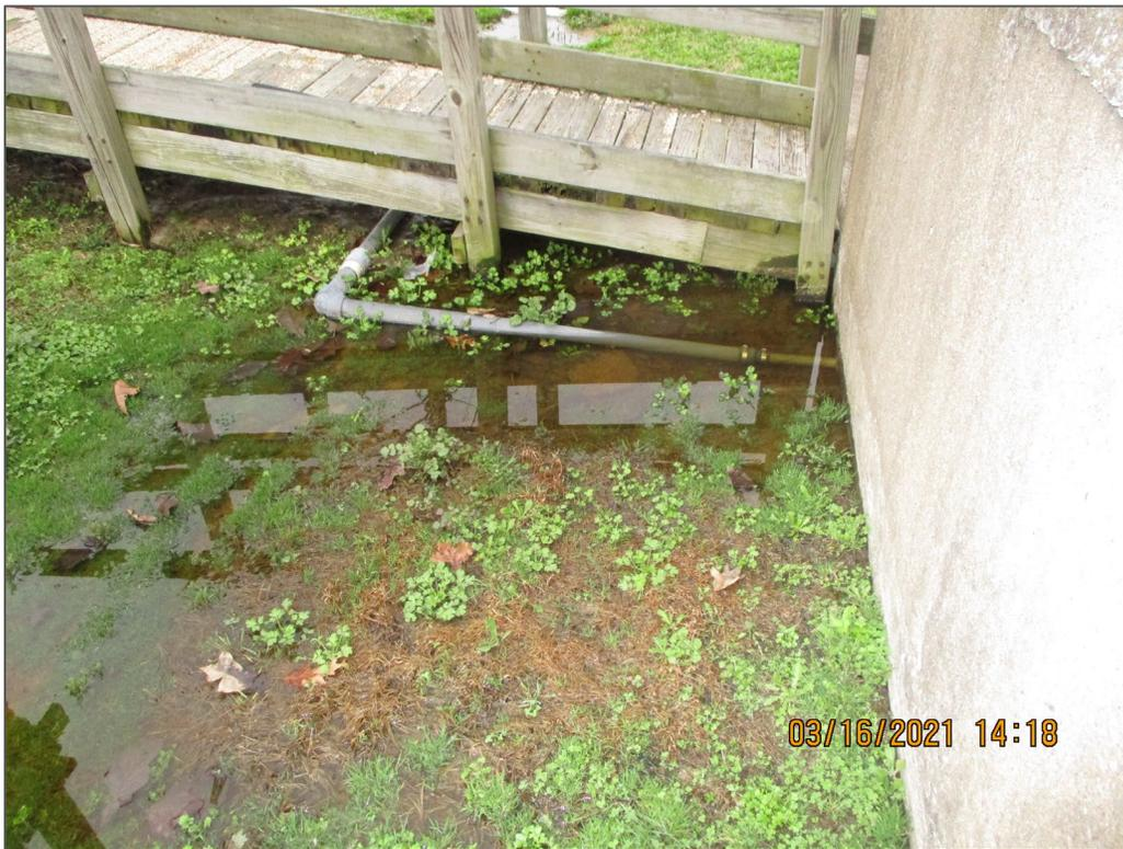
**Figure 9. Standing Water in the Surface Ditch near the Sump Pump Discharge**
