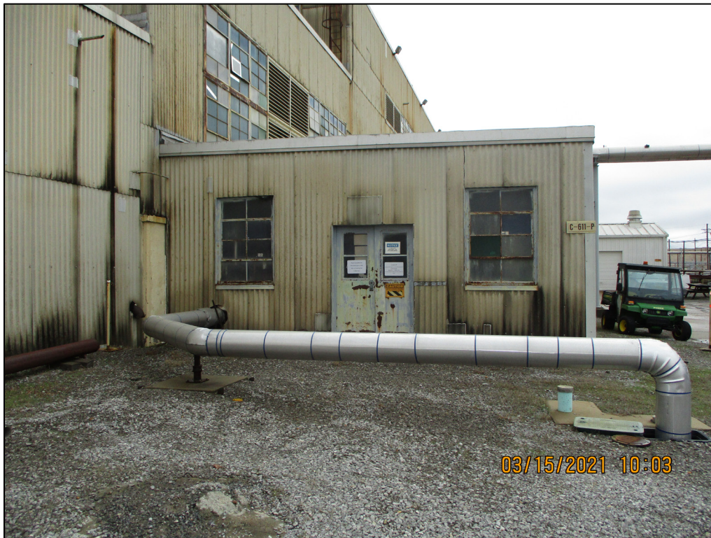
Figure 5. Exterior View of the West Side of C-611-P (Looking East)
