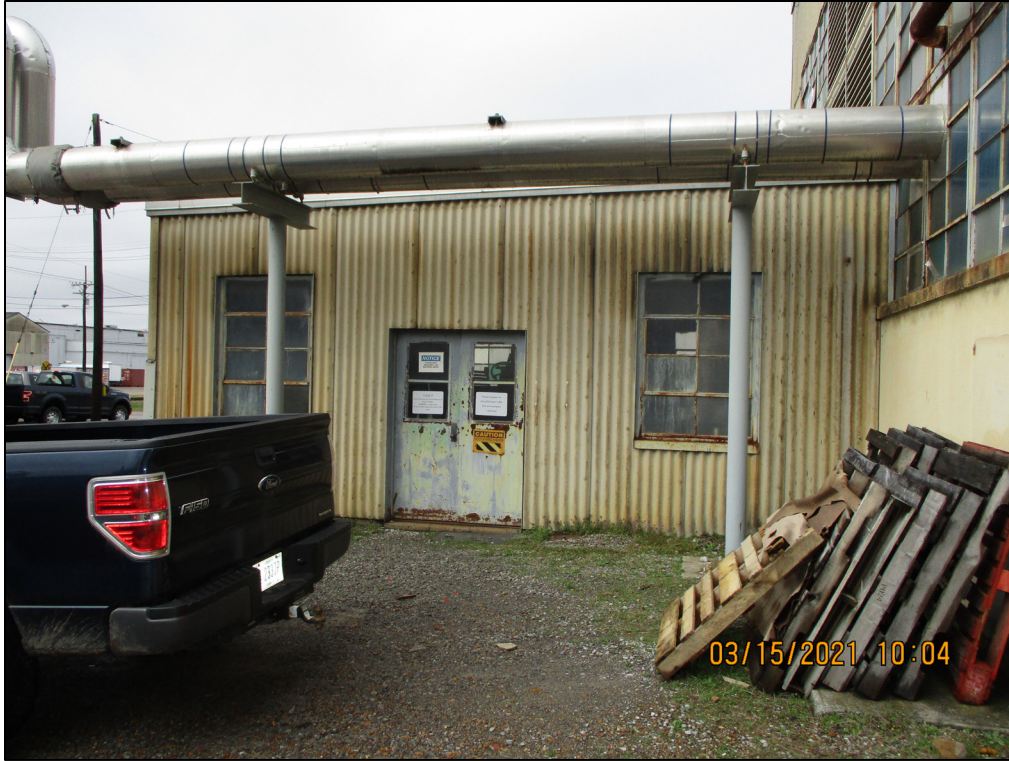
Figure 4. Exterior View of the East Side of C-611-P (Looking West)
