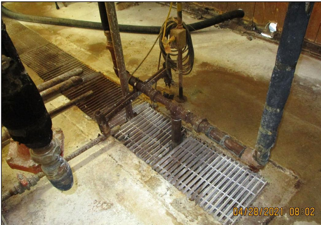
**Figure 36. Floor Trench with Suction Line in C-611-U**
