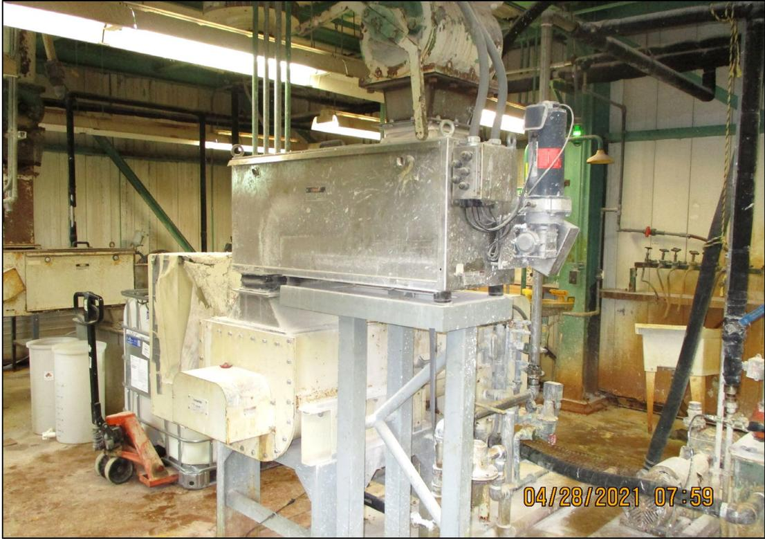
**Figure 35. Lime Feeder and Slaker in C-611-U**
