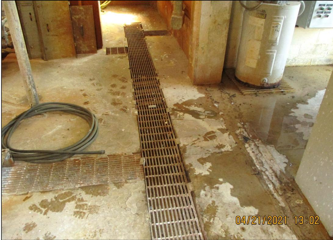
**Figure 13. Floor Collection Trench in C-611-B (Leads to an Exterior Sump Pit)**
