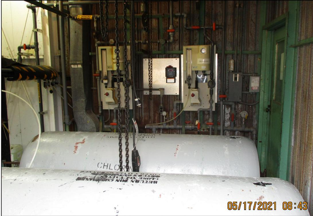
Figure 31. Chlorine Cylinders and Feeder Controls in C-611-S
