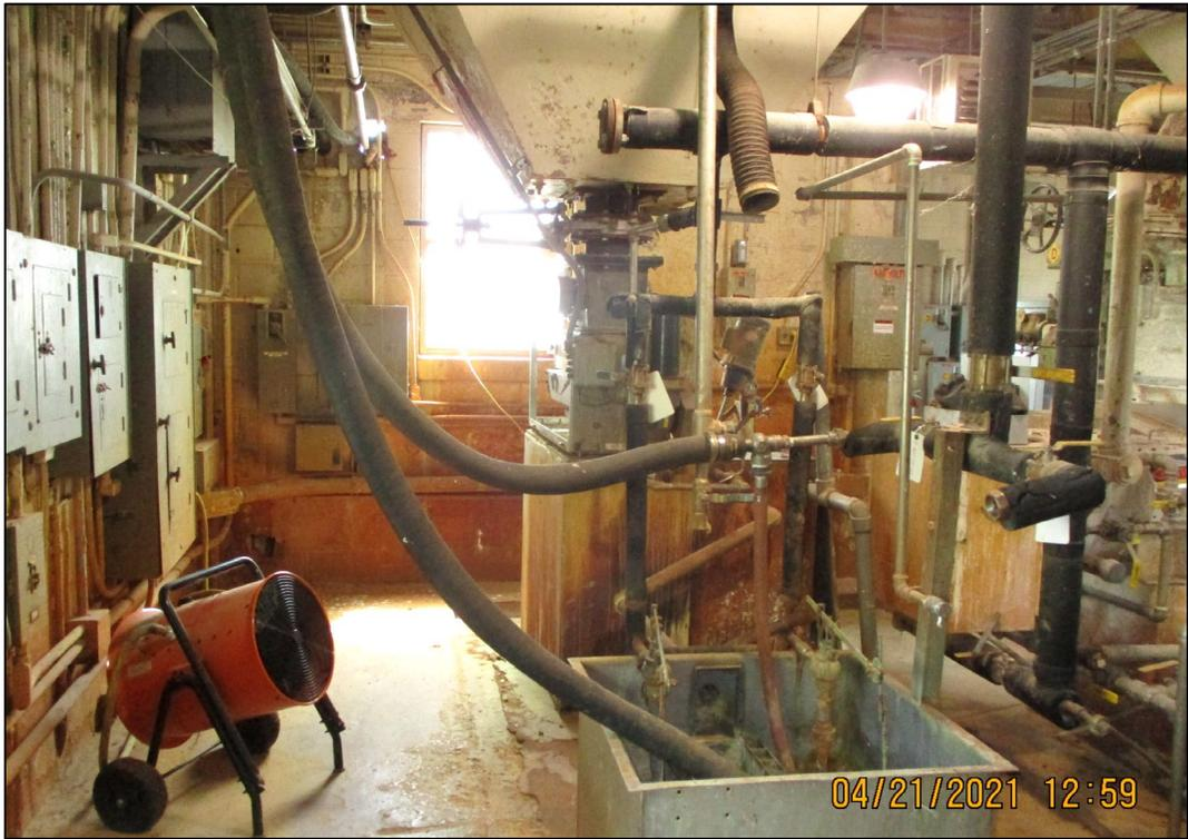
Figure 12. Ferric Sulfate Feeder System in C-611-B
