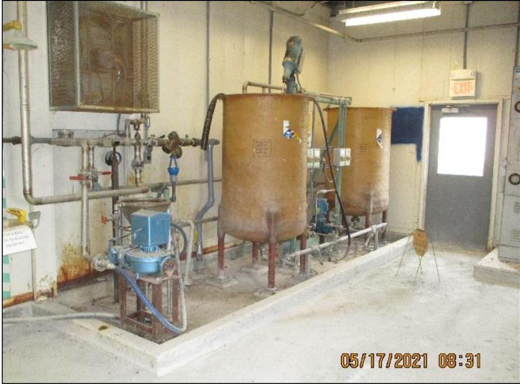
**Figure 19. Interior of C-611-F2 Showing Polymer Mixing Tanks**
