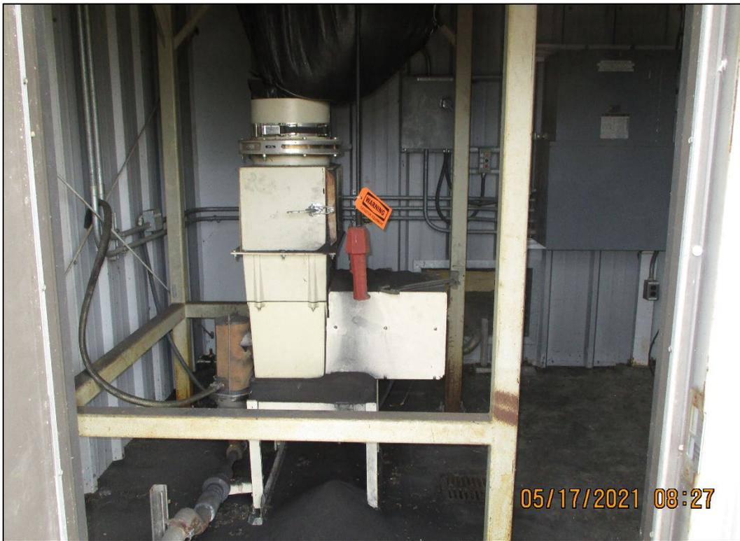
**Figure 20. Interior of C-611-F3 Showing the Activated Carbon Feeder**
