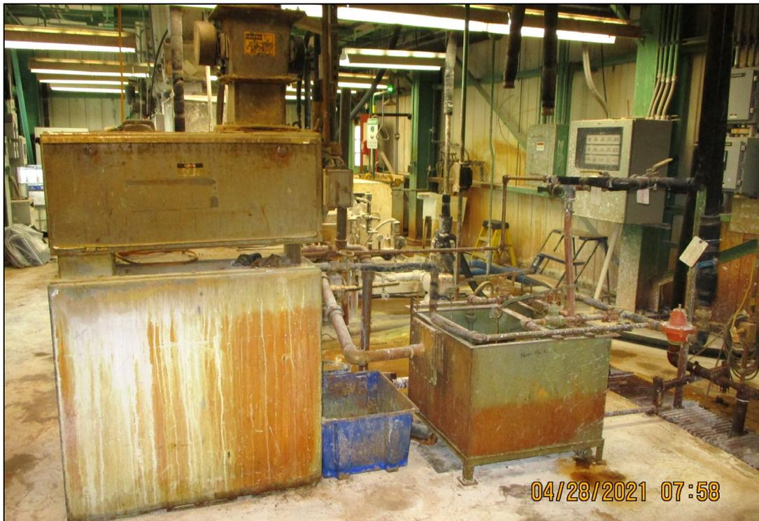
**Figure 34. Ferric Sulfate Feeder and Mixing Tank in C-611-U**
