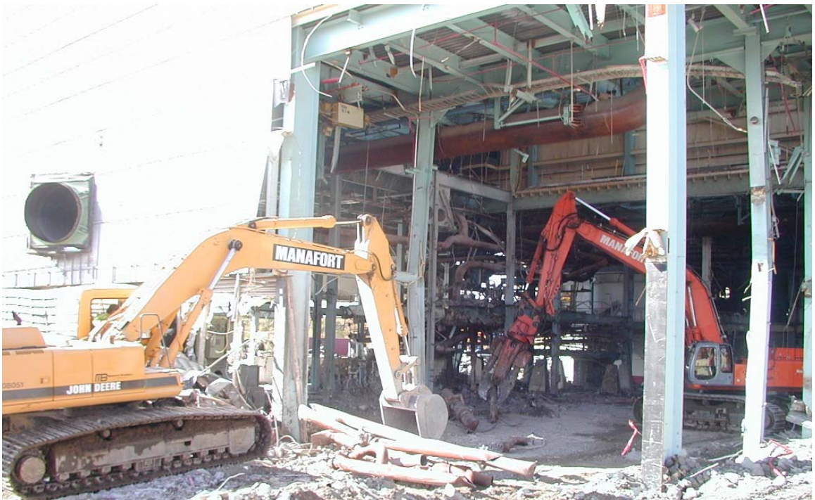
Figure A.4. Interior Building Mezzanine and Equipment Removal Prior to Demolishing the Structure
