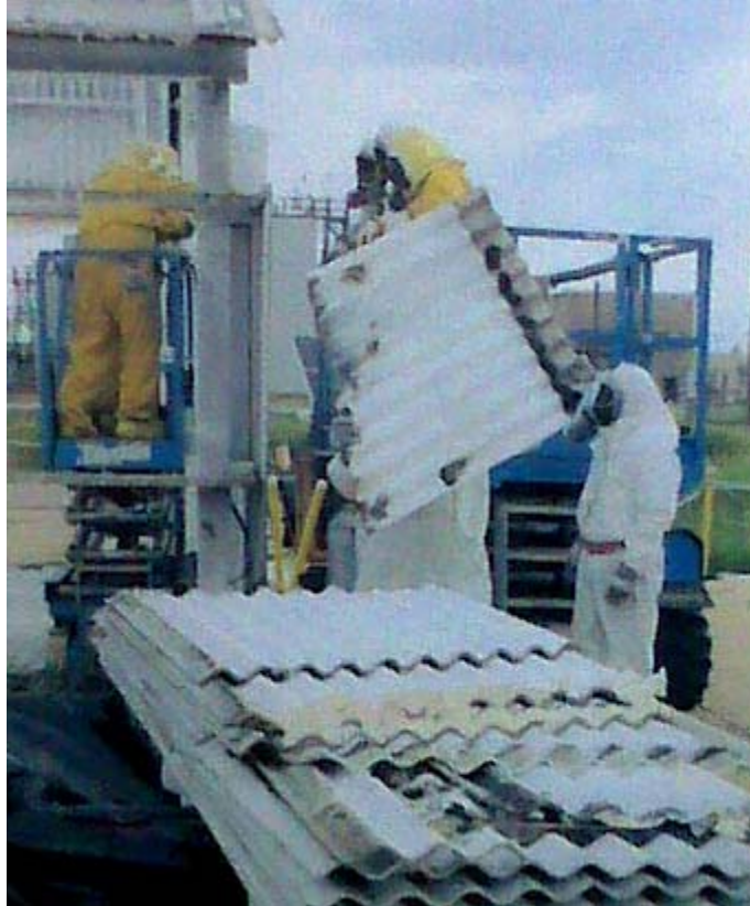
Figure A.5. Transite Siding Removal and Packaging
