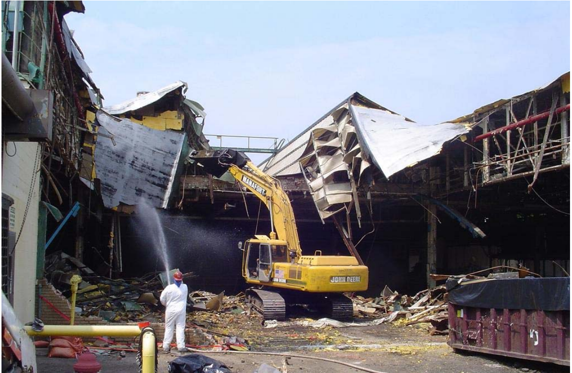
Figure A.3. Building Structure and Roof Demolition (Shear and Fugitive Dust Control)
