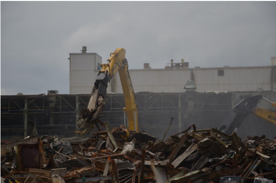
Figure A.7. Downsizing Debris from C-410 Demolition
