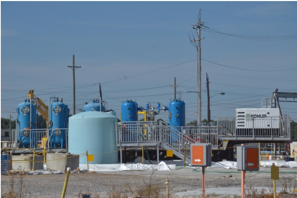
Figure A.15. Water Treatment System Used to Treat Water for Discharge from Zone 26 Basement
