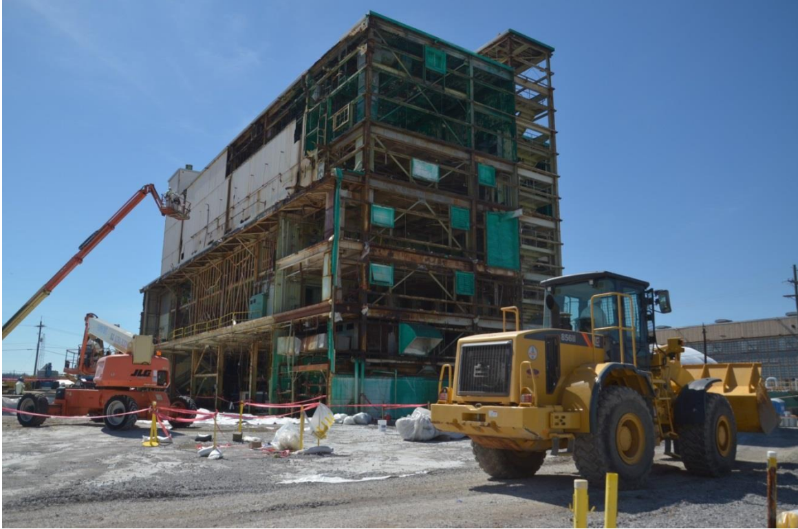
Figure A.6. Transite Removal from East Wall of C-420 Building (view toward southwest)
