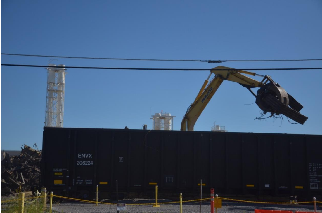
Figure A.12. C-410 Demolition Debris Loading into Gondolas (view toward north)
