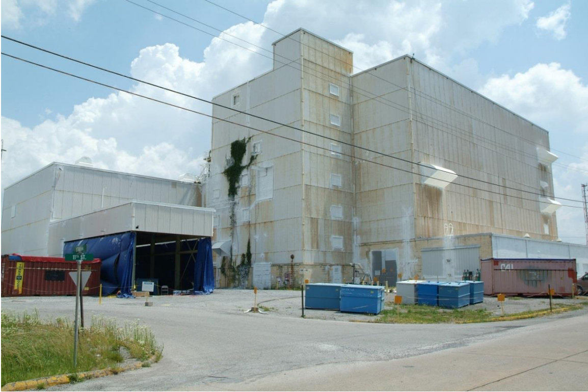
Figure A.1. C-410 Complex Prior to Demolition (view toward southeast)
