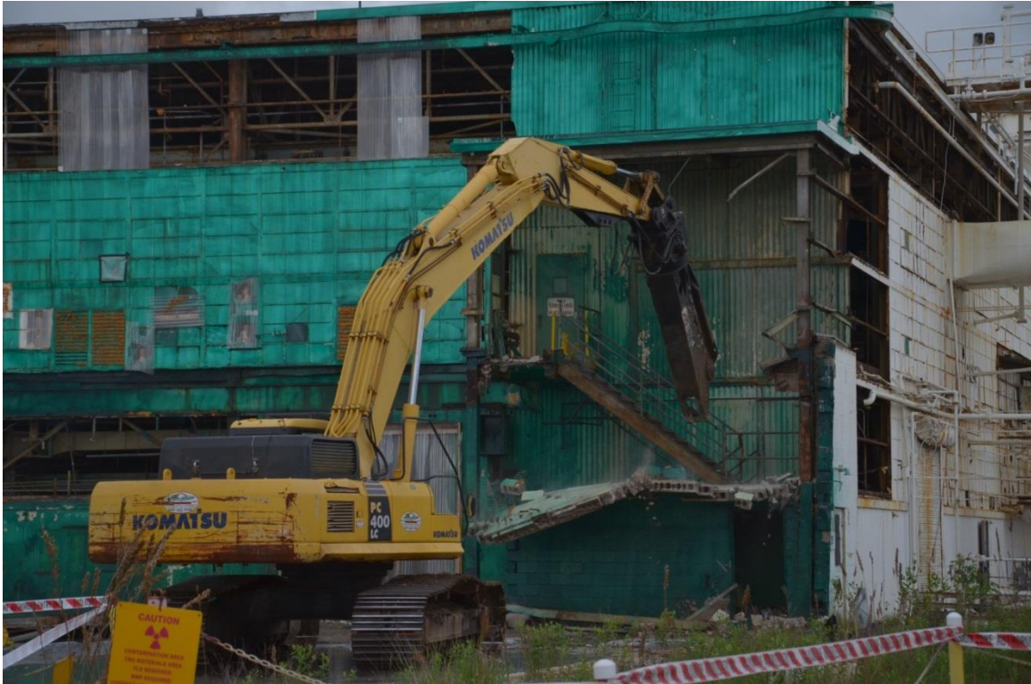
Figure A.3. Demolition of C-410 Original Feed Plant (view toward east)
