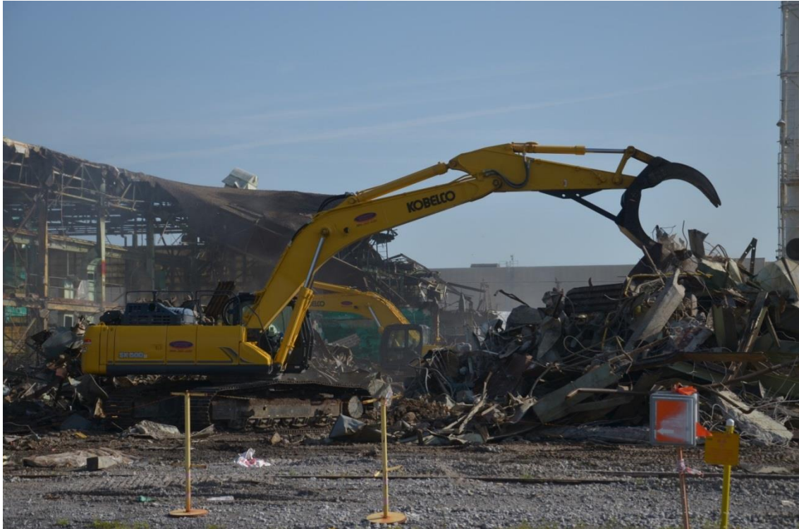
Figure A.10. Downsizing and Segregation of Demolition Debris
