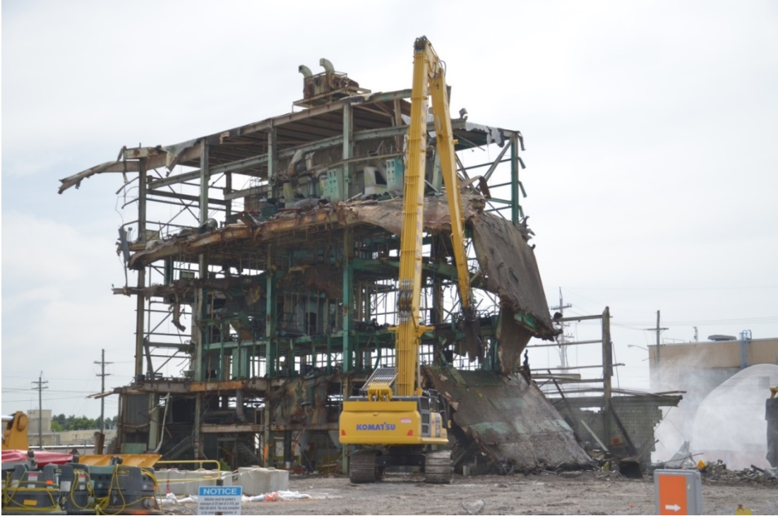
Figure A.14. High Reach Excavator Demolishing Northern End of C-420 Building (view toward southwest)
