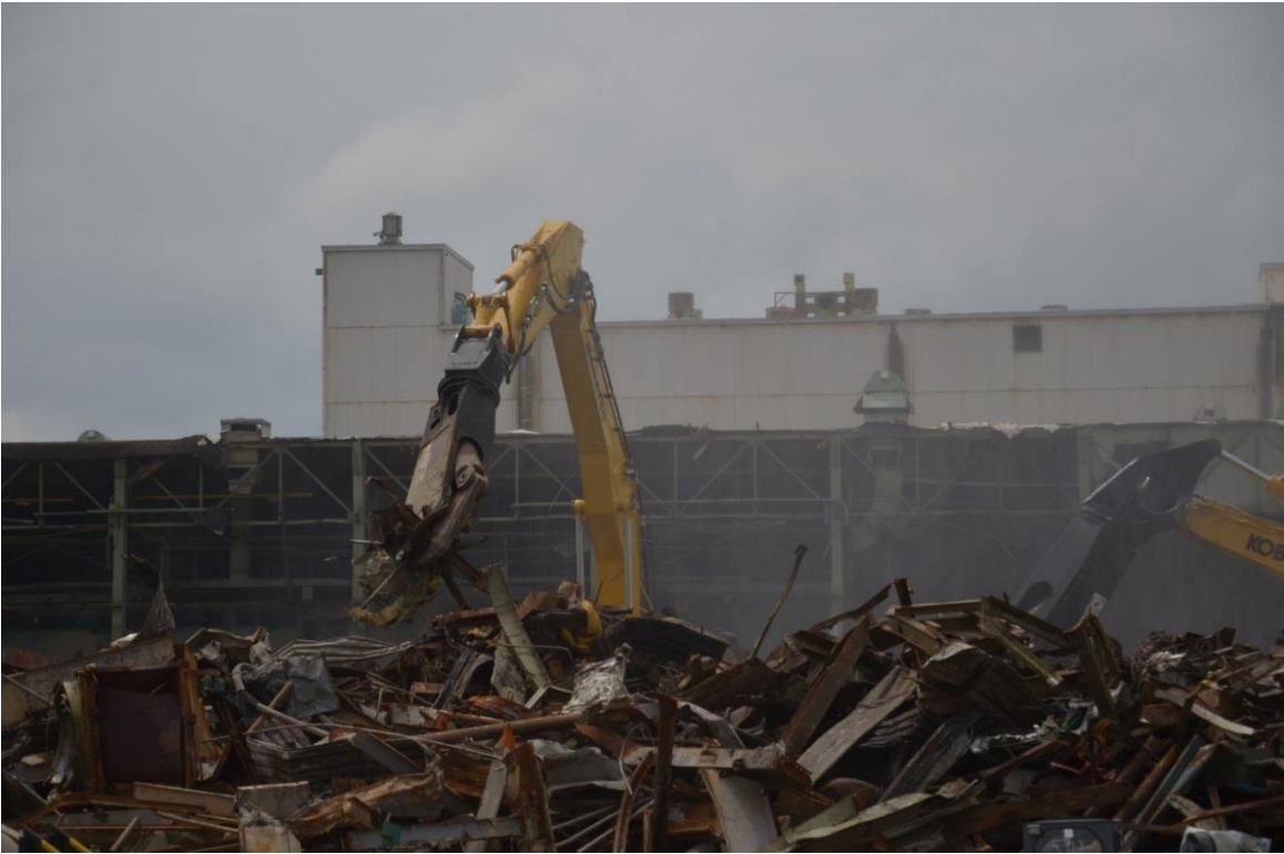
Figure A.7. Downsizing Debris from C-410 Demolition
