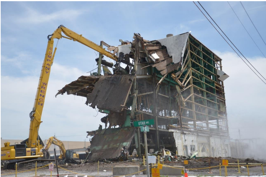
Figure A.13. High Reach Excavator Demolishing Northern End of C-420 Building (view toward southeast)
