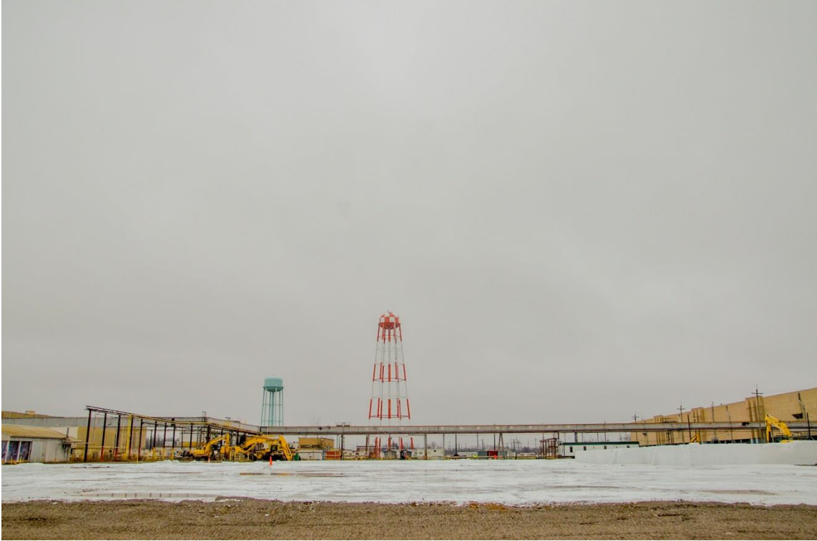
Figure A.16. C-410 Slab in Final State with Epoxy Coating Applied (view toward plant east)
