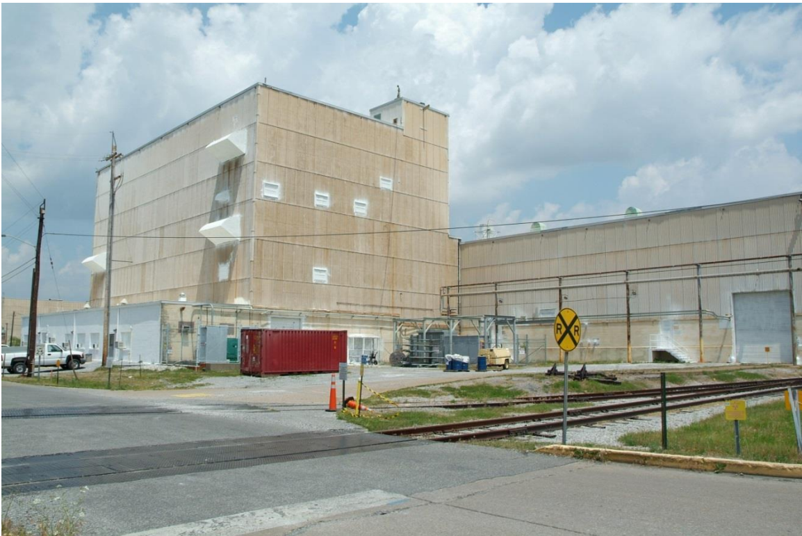
Figure A.2. C-410 Complex before Demolition (view toward northeast)
