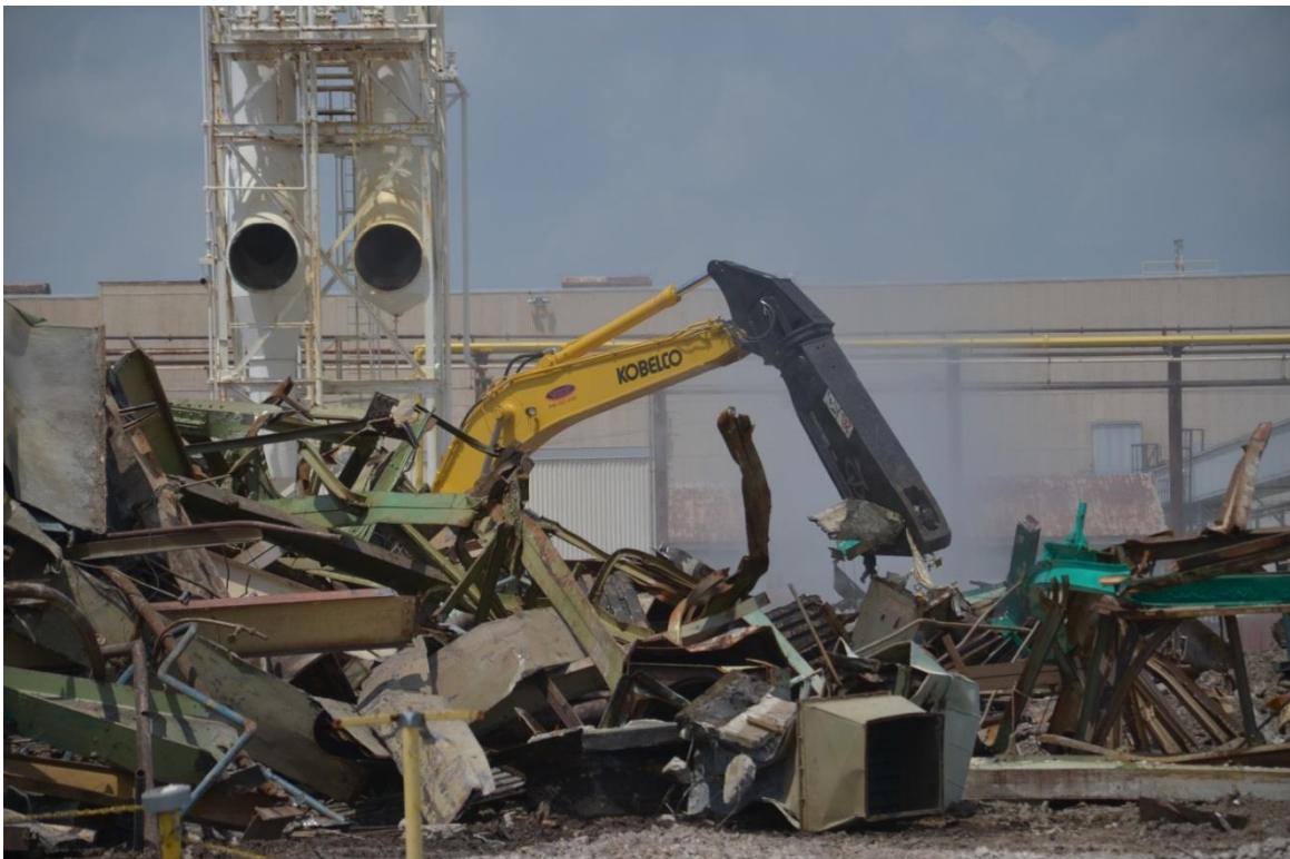
Figure A.11. Downsizing Demolition Debris (view toward north)
